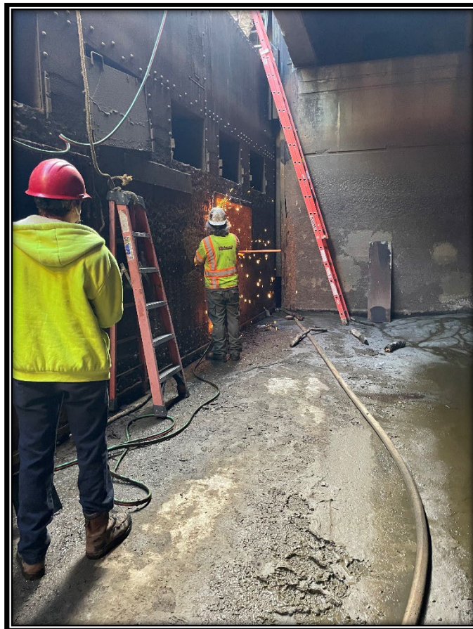
Figure:1 Driscoll Construction prepping tide gate for removal.
