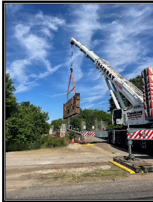
Figure 2: Driscoll Construction removed tide gate.
