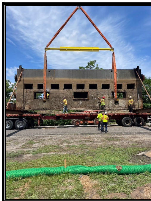
Figure 3: Driscoll Construction moved to staging area.
