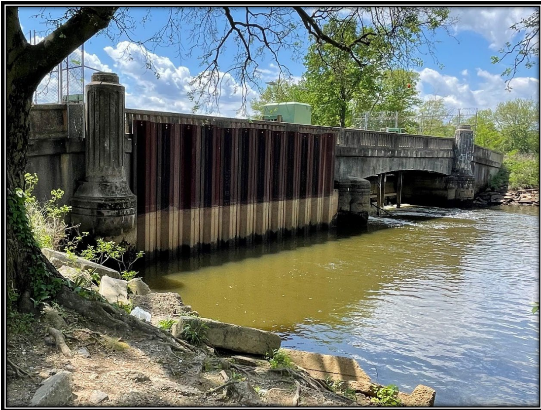
Figure:1 Kaighn Avenue Dam – East Tide Gate.
