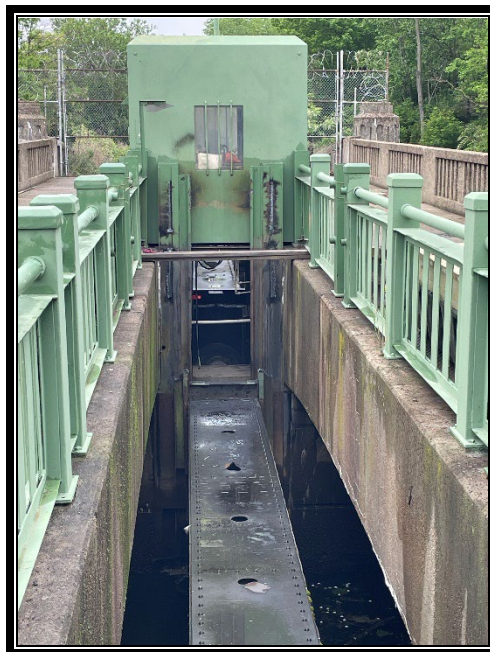
Figure 3: Driscoll Construction removed both lift assemblies and lift cylinders.
