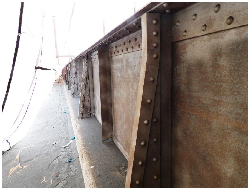
Looking south along the west girder after blasting
