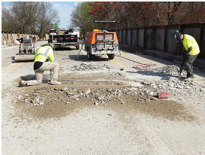
Workers continued removing deteriorated deck concrete
