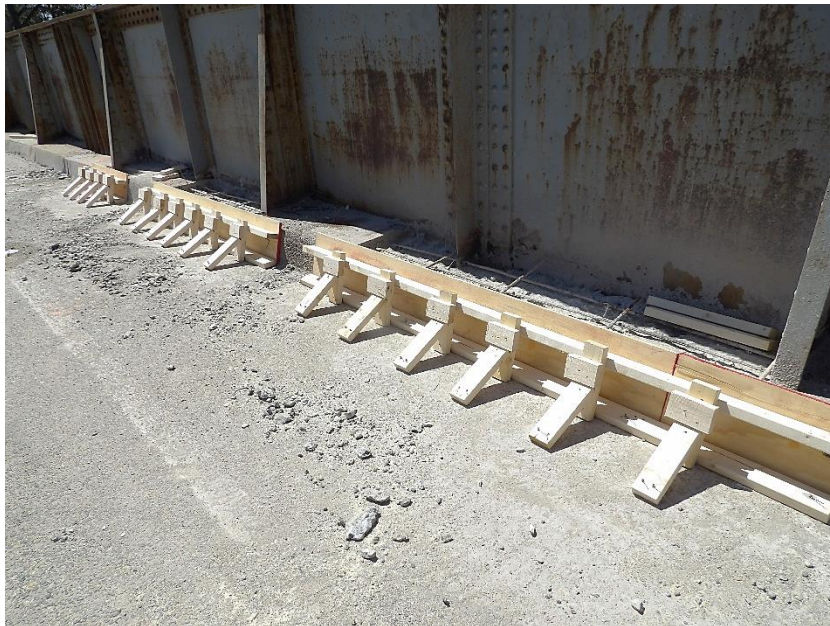
Workers installed forms for the new bridge curb sections
