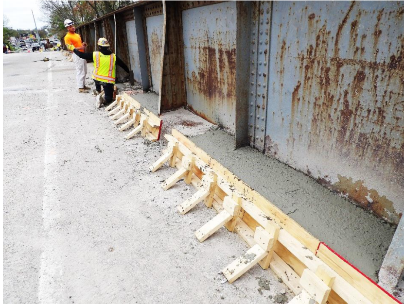
Workers formed and poured portions of the bridge curbs
