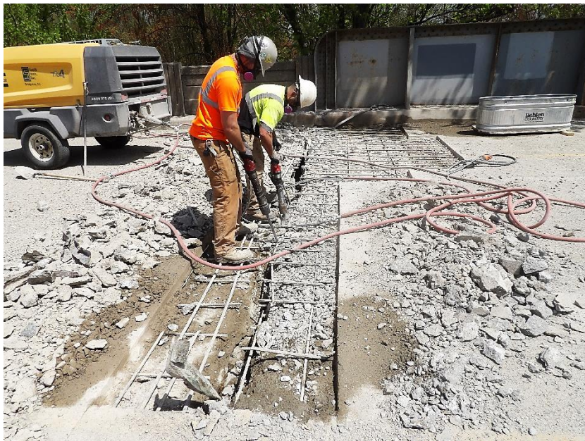
Workers began demolition of the north abutment deck joint
