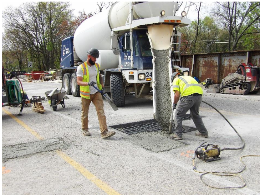
Workers poured concrete in the open patch areas
