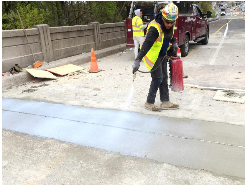
Workers sprayed all fresh concrete with a curing compound
