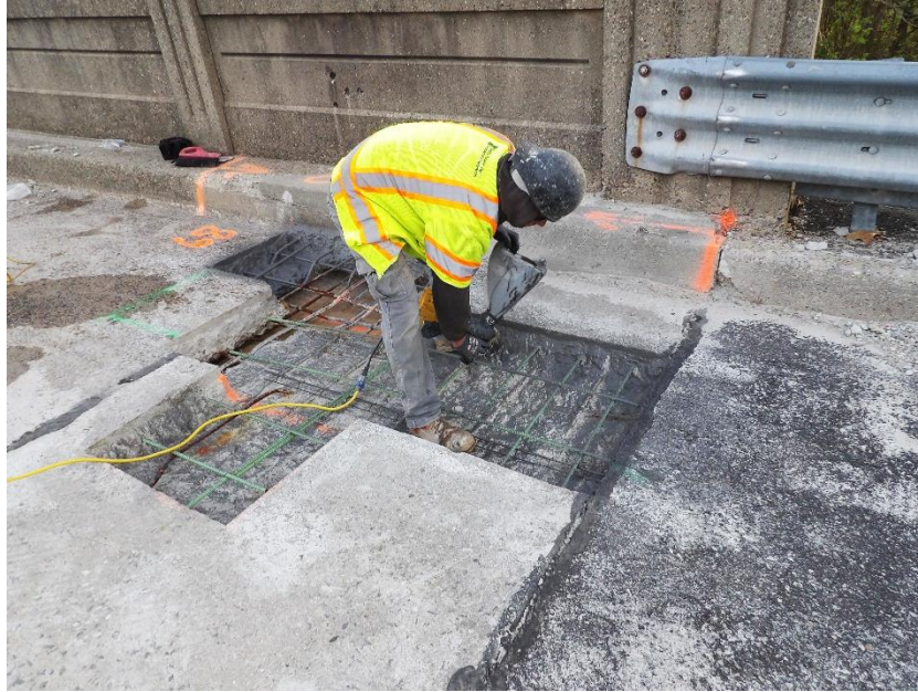
Workers prepared deck patch areas for new concrete
