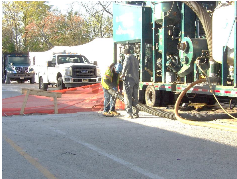
Workers assembling the dust vacuum line
