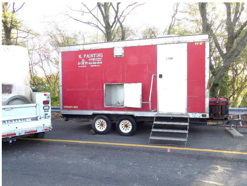
On-site lead decontamination shower
