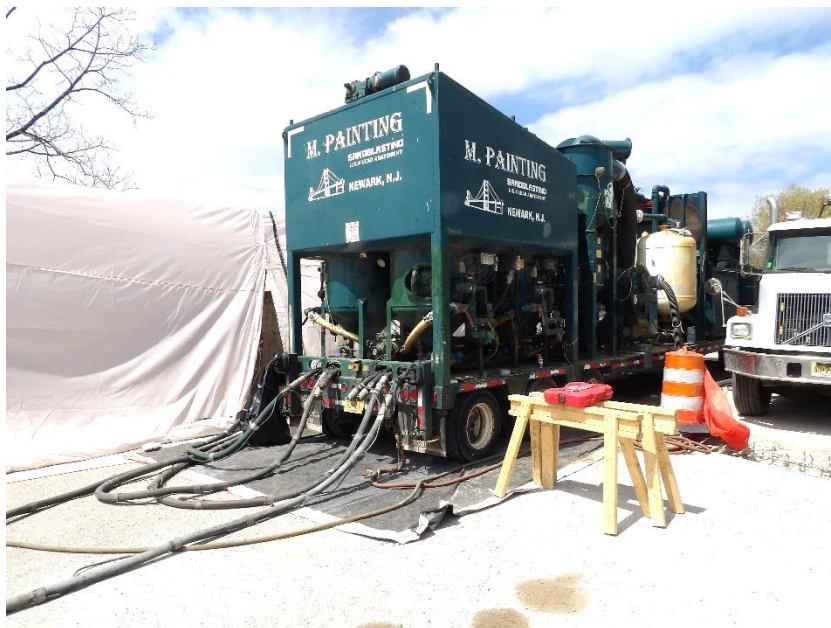
Workers set-up the sand blasting and power units
