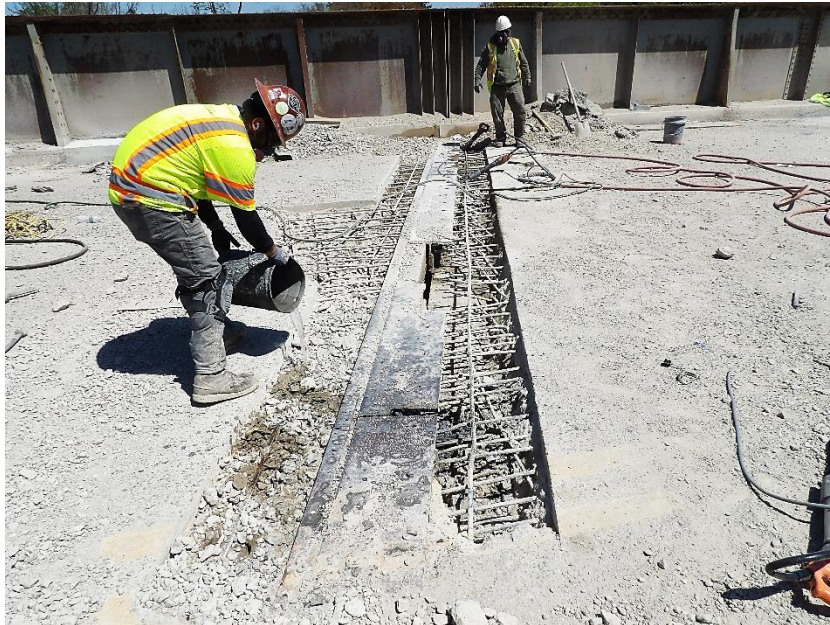
Workers began demolition of the center pier deck joint
