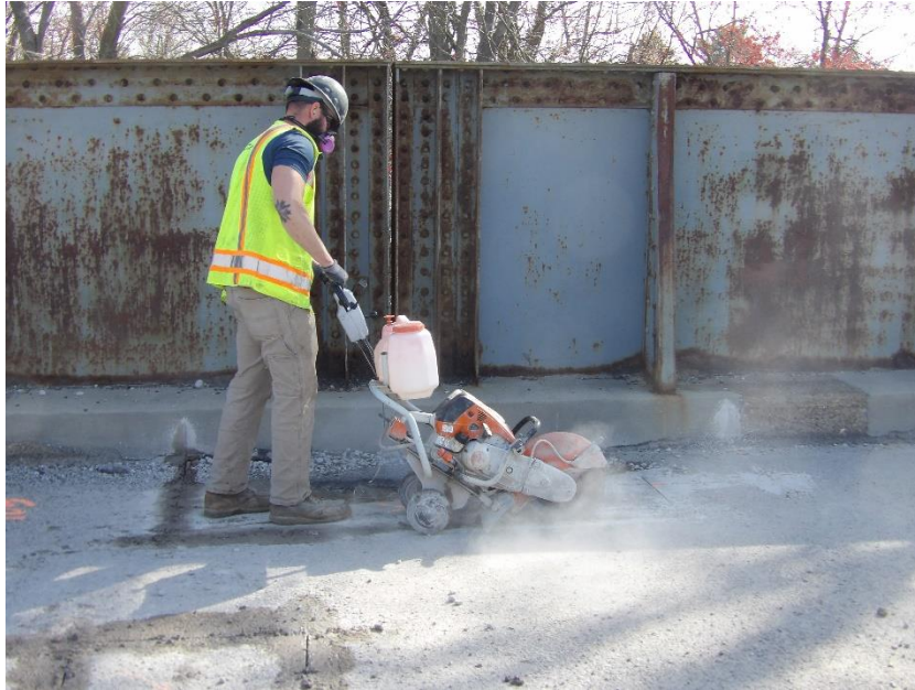
Photo 6 – Saw-cutting around deteriorated deck areas continued
