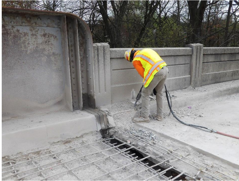
Photo 8 – Workers began demolition of deteriorated bridge curbs
