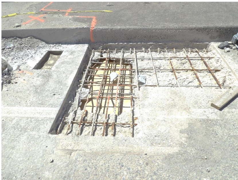
Photo 5 – Workers install formwork prior to pouring new concrete
