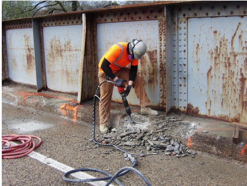
Photo 10 – Workers continued chipping deteriorated curb concrete
