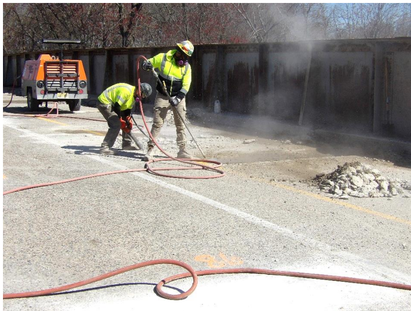
Photo 3 – Workers cleaned patch areas with compressed air
