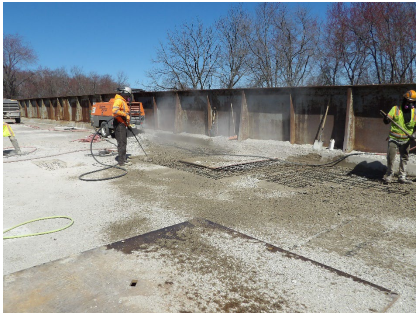
Photo 9 – Concrete chipping and debris removal continued all week
