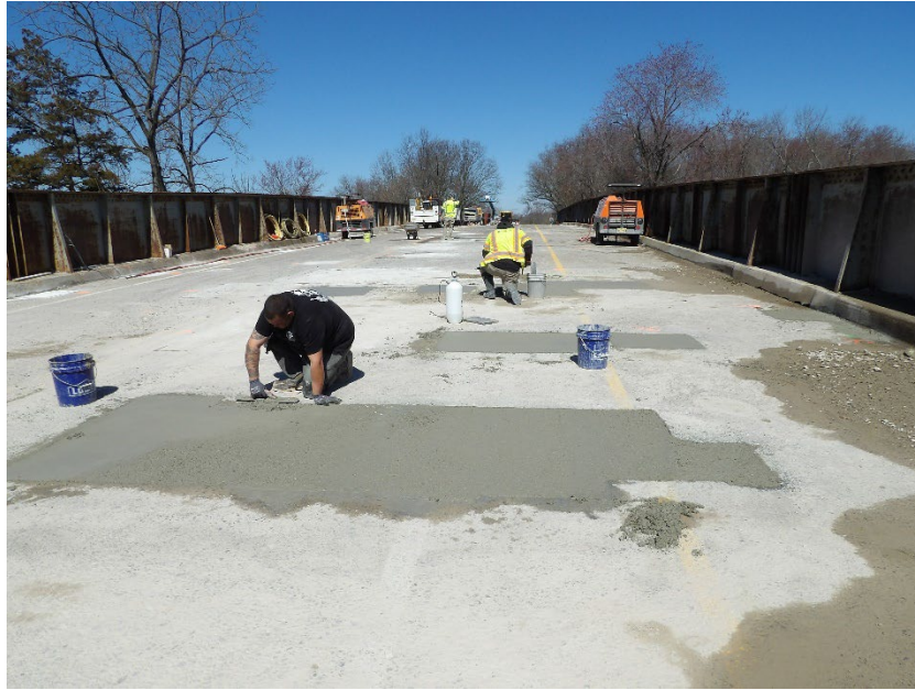
Photo 8 – Resident Engineer and worker completed sounding the entire deck for repairs
