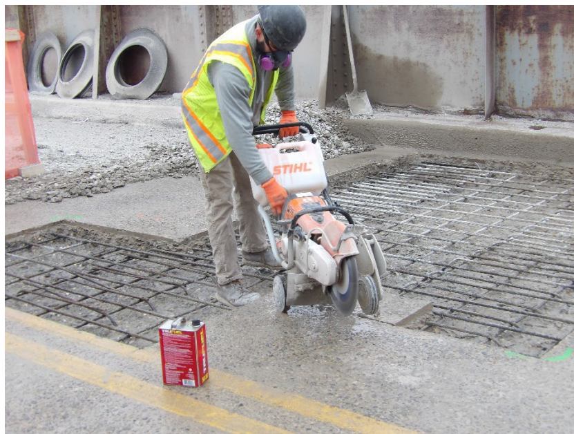
Photo 7 – Concrete cutting and removal continued throughout the week
