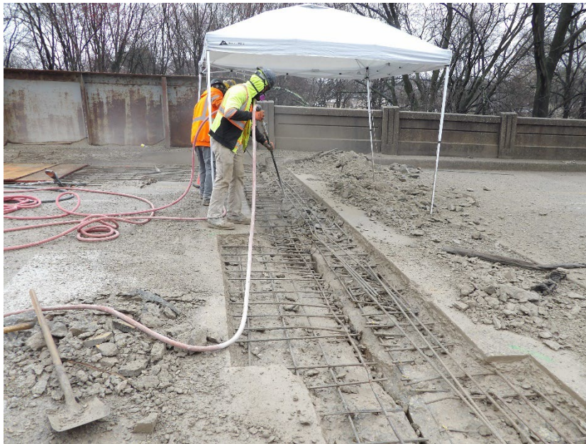
Photo 11 – Workers resumed demolition work on the south abutment deck joint
