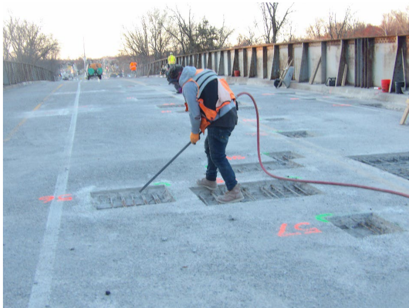
Photo 3 – Workers cleaned patch areas
