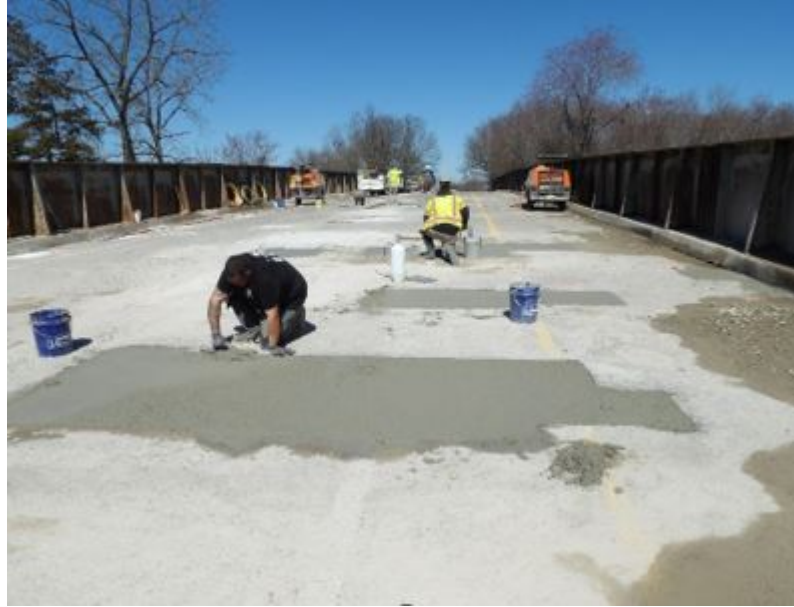
Photo 10 – Workers poured the 3 rd round of concrete in open patch areas
