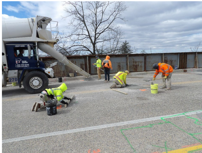
Photo 5 – Workers poured and finished the concrete deck patches
