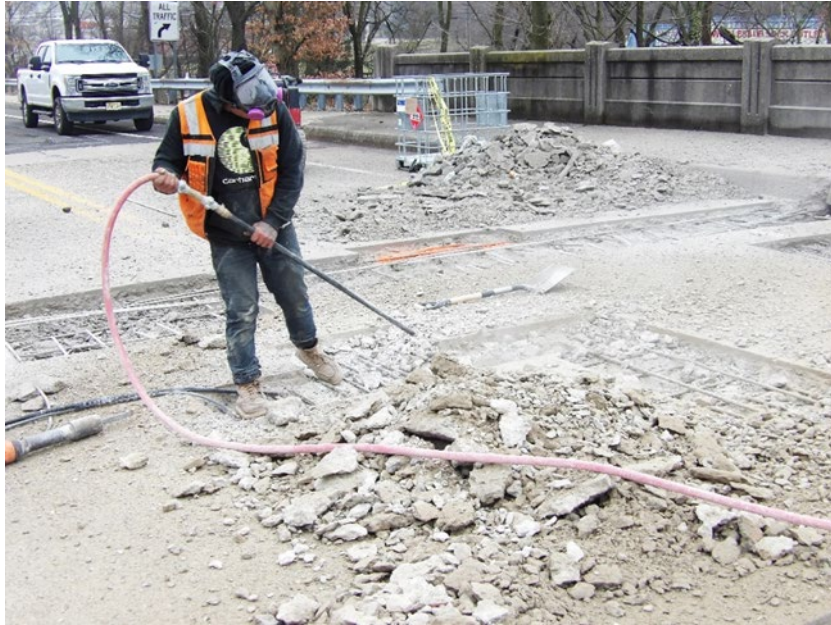
Photo 4 – Workers began demolition of the south deck join
