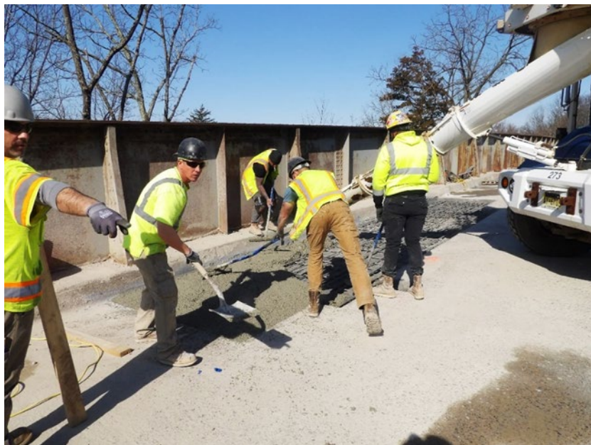
Photo 10 – Workers poured concrete in open patch areas
