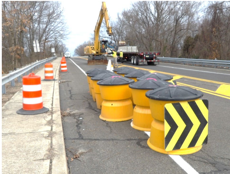
Photo 1 – Contractor began mobilization and set-up traffic control, closing Haddon Avenue southbound
