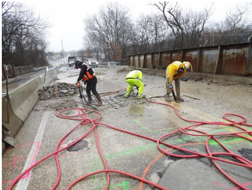
Photo 3 – Workers saw-cut areas and began concrete removal.
