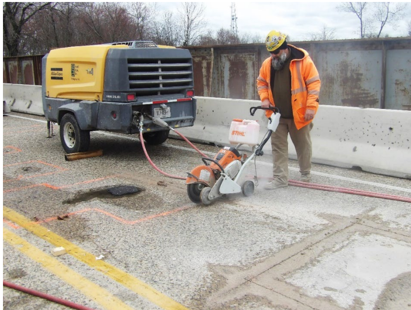
Photo 4 – Workers began demolition of the south deck join
