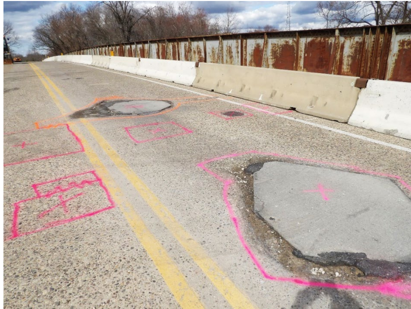
Photo 2 – Resident Engineer located and marked out deteriorated concrete for removal
