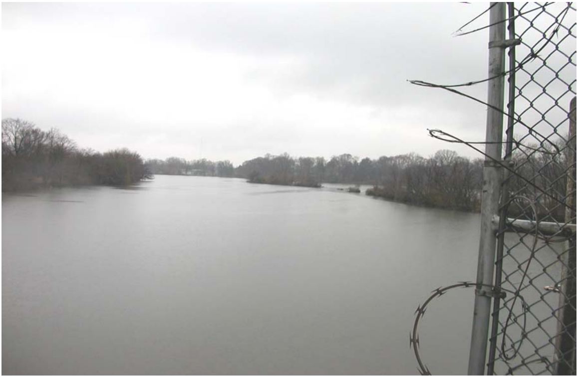
View on the Cooper River Lake from the Cooper River Parkway Dam
