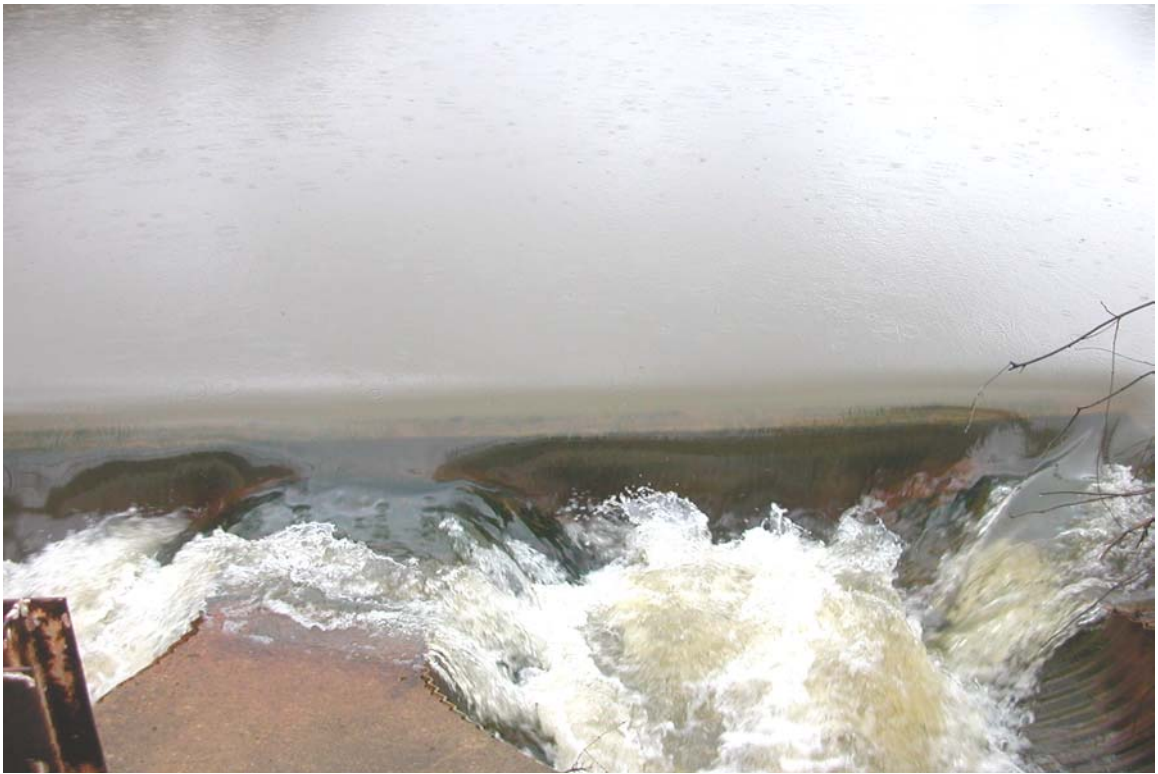
Wallworth Lake Dam, View from the bridge - Wallworth Park in Haddonfield
