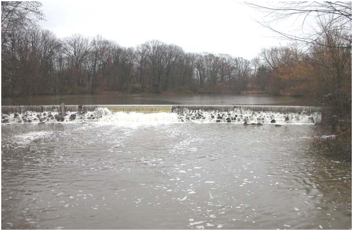
Spill through the Evans Pond Dam to Wallworth Lake
