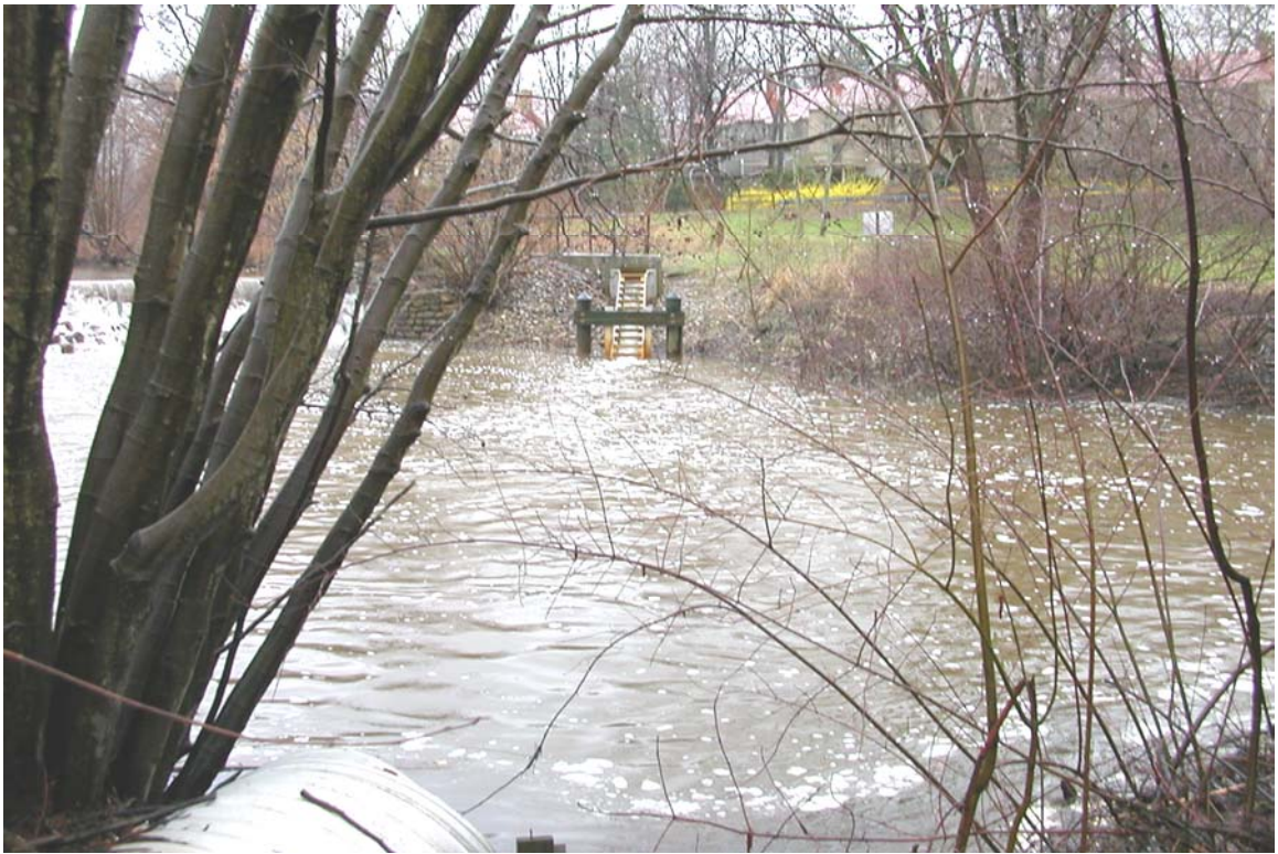
Wallworth Lake: Fishway from Wallworth Lake to Evans Pond, at the bottom of the picture, stormwater discharge. North side of the lake
