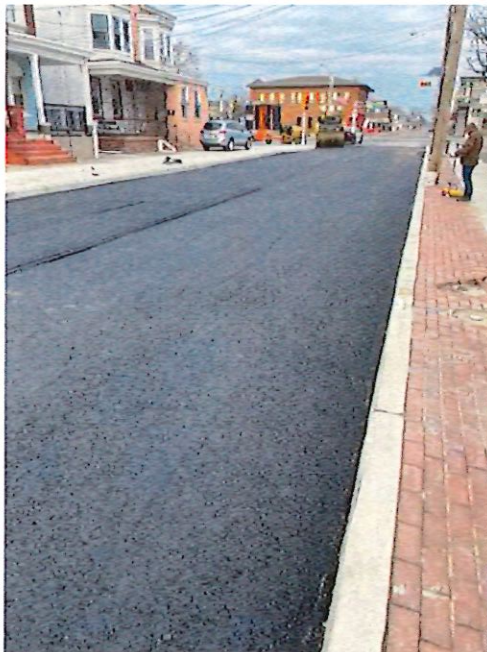
Figure 4: Compacting HMA Base Course
