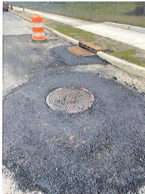
Figure 5: Resetting Manhole Casting
