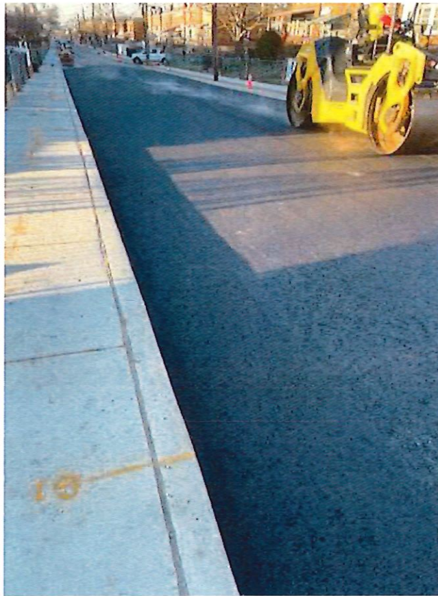
Figure 1: Compacting HMA Base Course
