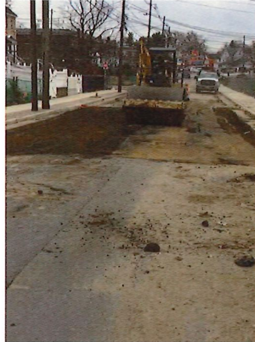
Figure 3: Compacting Roadway Subbase
