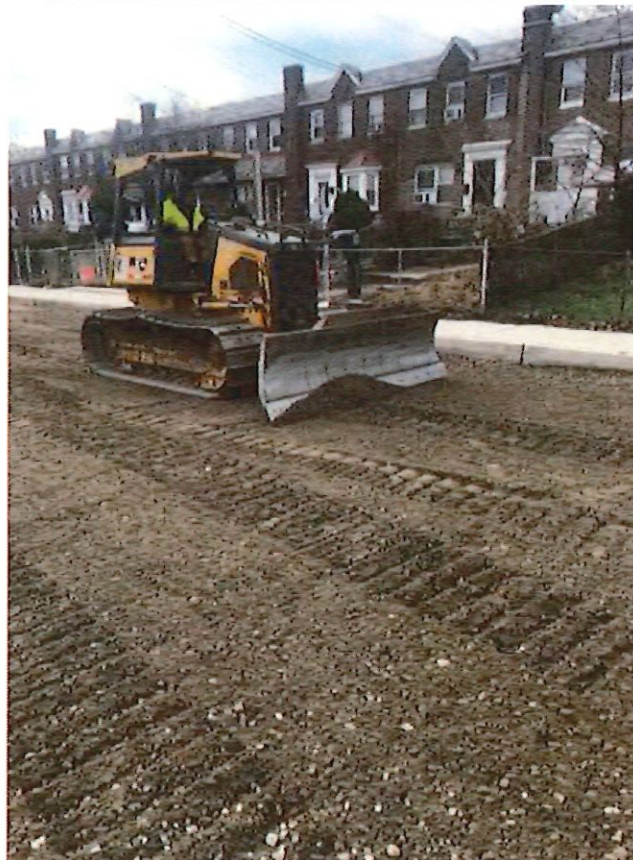
Figure 1: Leveling DGA Base Course
