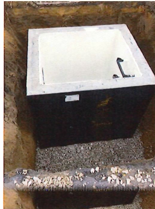
Figure 5: Installing Inlet Type, B
