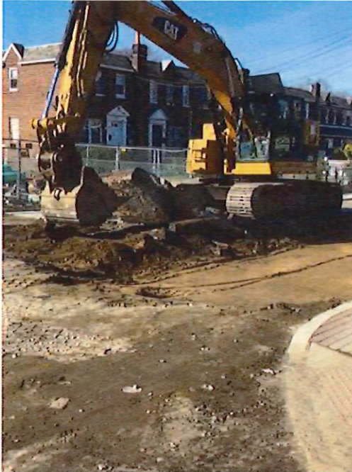
Figure 2: Excavating Existing Roadway
