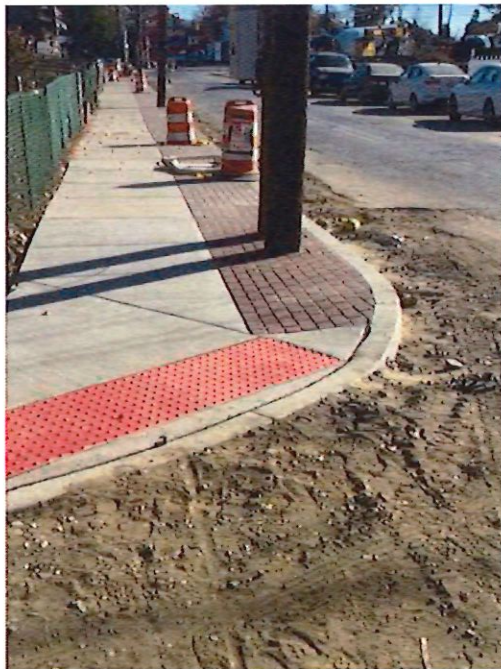
Figure 4: ADA Ramp and Brick Pavers
