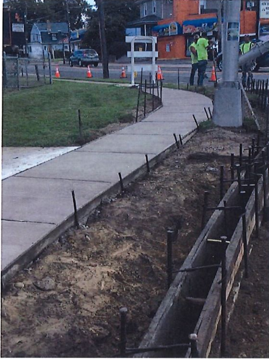
Figure 2: Concrete Sidewalk & Forming Curb
