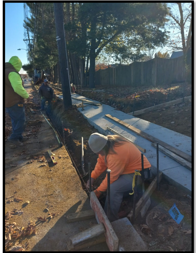
Photograph 2 – Setting forms for concrete curb pour.
