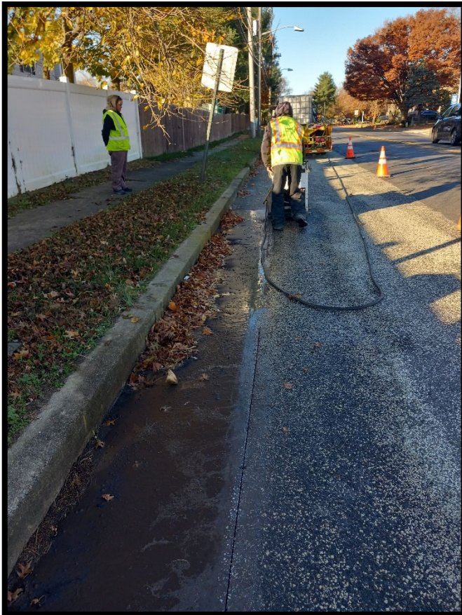
Photograph 1 – Concrete crew sawcutting to remove asphalt for concrete curb replacement.
