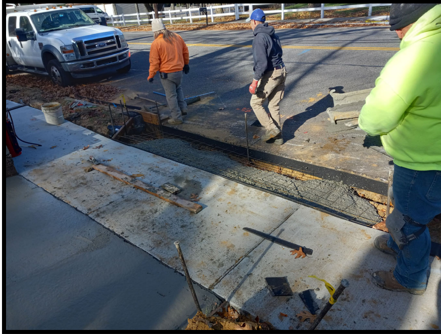
Photograph 5 – Concrete crew installing driveway apron with welded wire fabric reinforcement.
