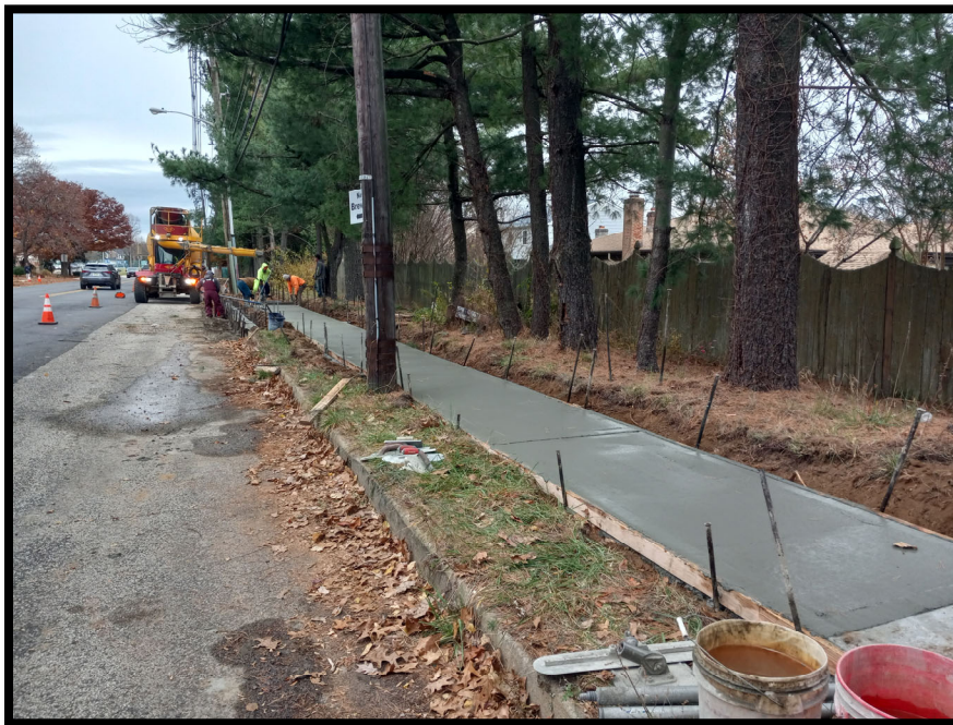
Photograph 6 – Concrete crew installing new sidewalk.
