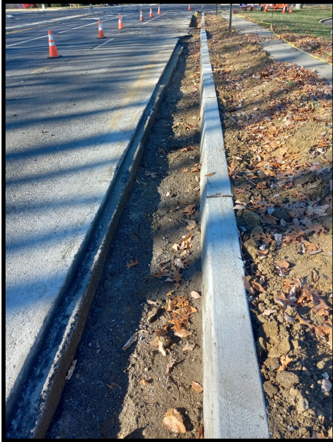
Photograph 3 – New concrete curb installed and preparation for asphalt restorations underway.
