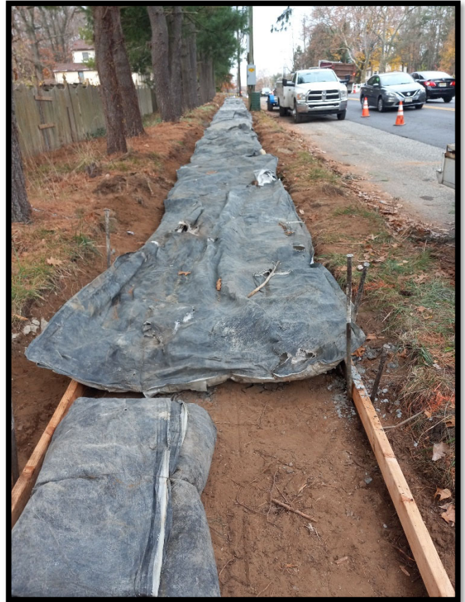
Photograph 8 – Concrete blankets used overnight to protect fresh concrete from freezing.
