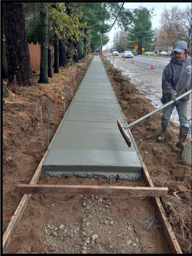
Photograph 7 – Broom finish being applied to newly poured concrete sidewalk.
