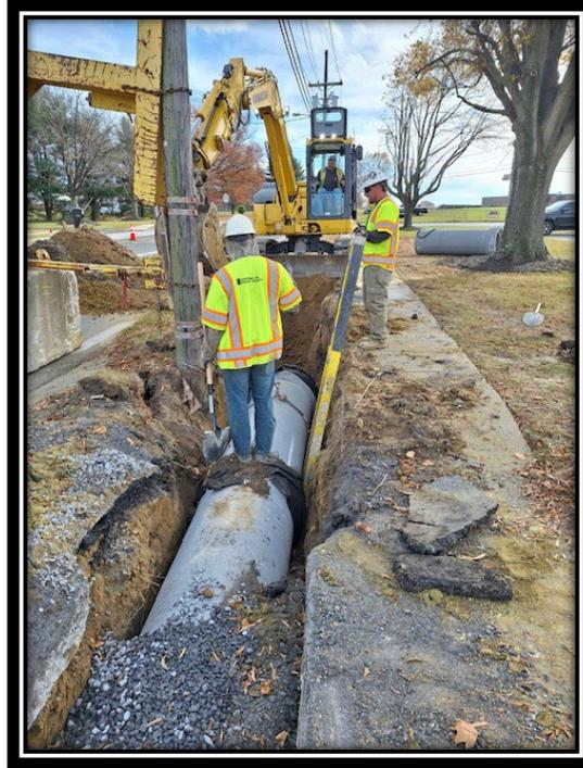
*Figure: 2 – Installation of 18” RCP along the southbound lane between Chews Landing Road and Seabury Drive*
