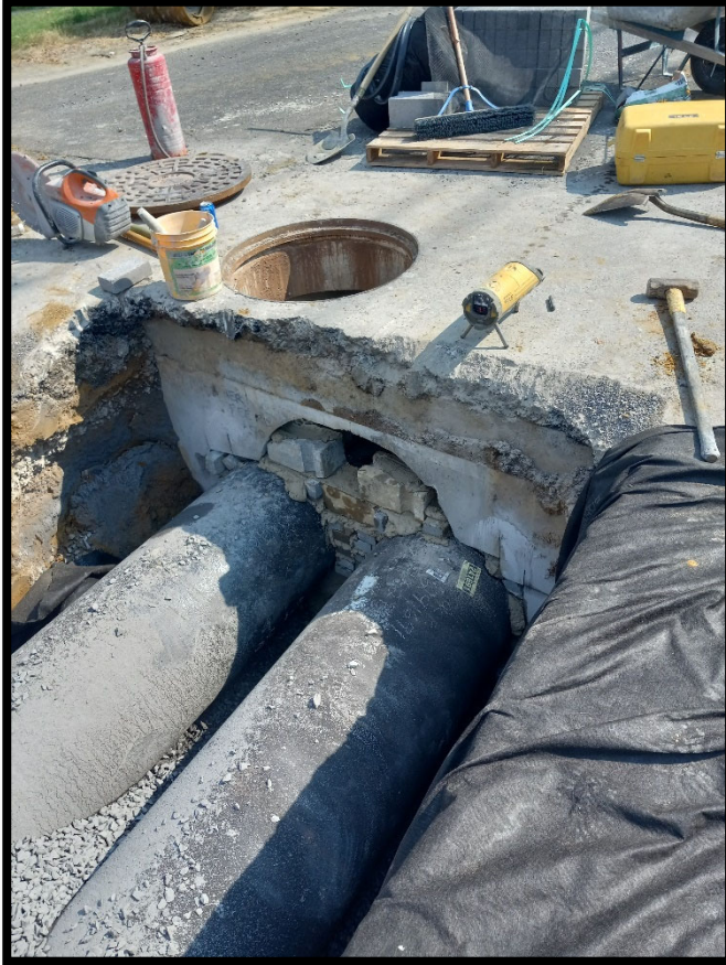
Photograph 3 – Dual 24” Ductile Iron Storm Pipe connection at Diverter Manhole.
