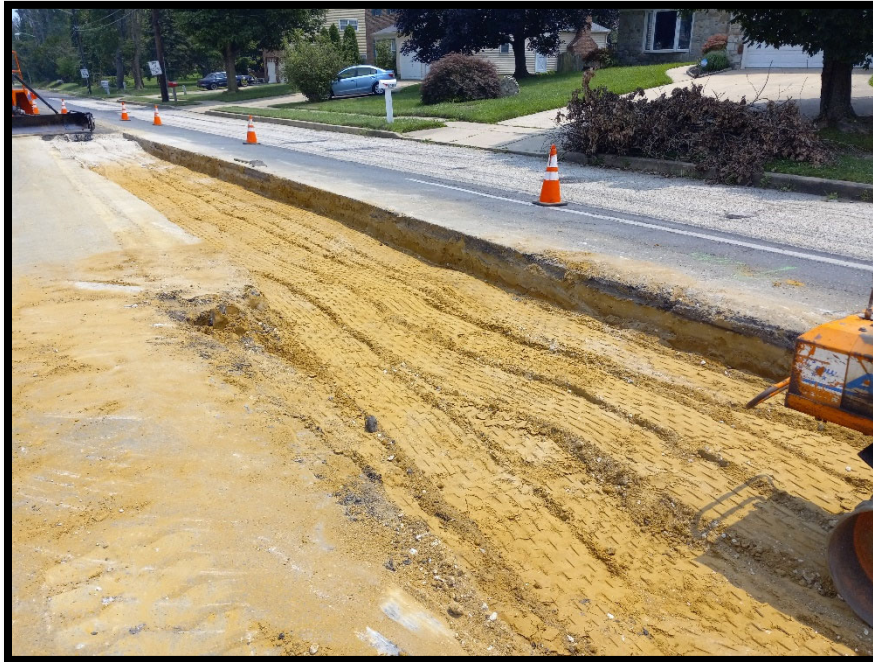
Photograph 3 – Trench restoration after installation of 15" RCP storm pipe.
