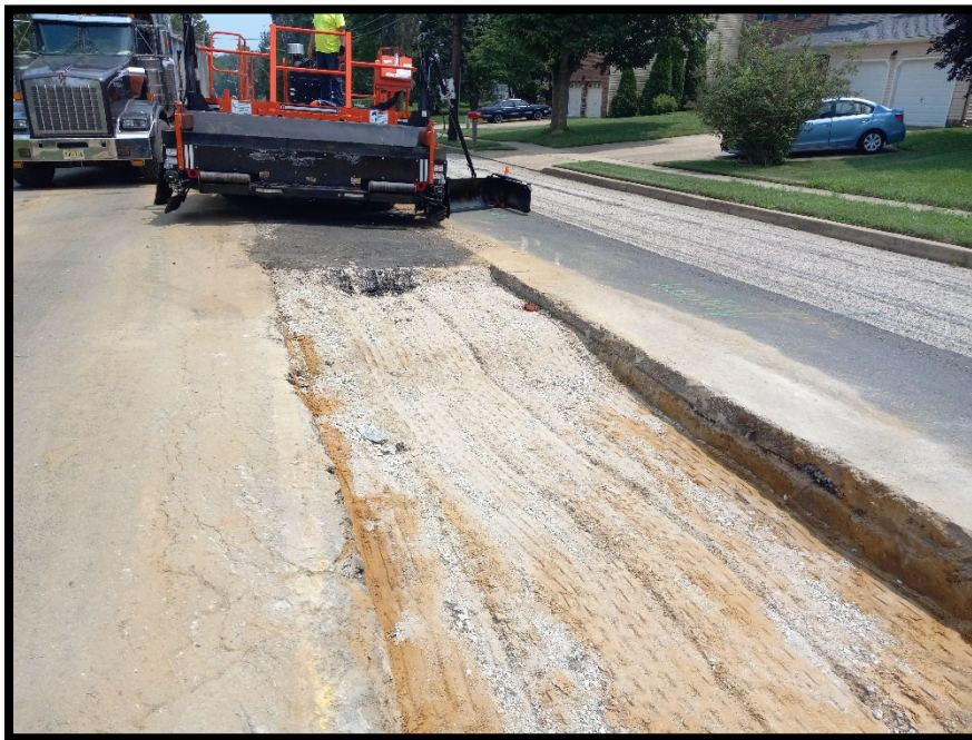
Photograph 4 – Trench restoration after installation of 15" RCP storm pipe.
