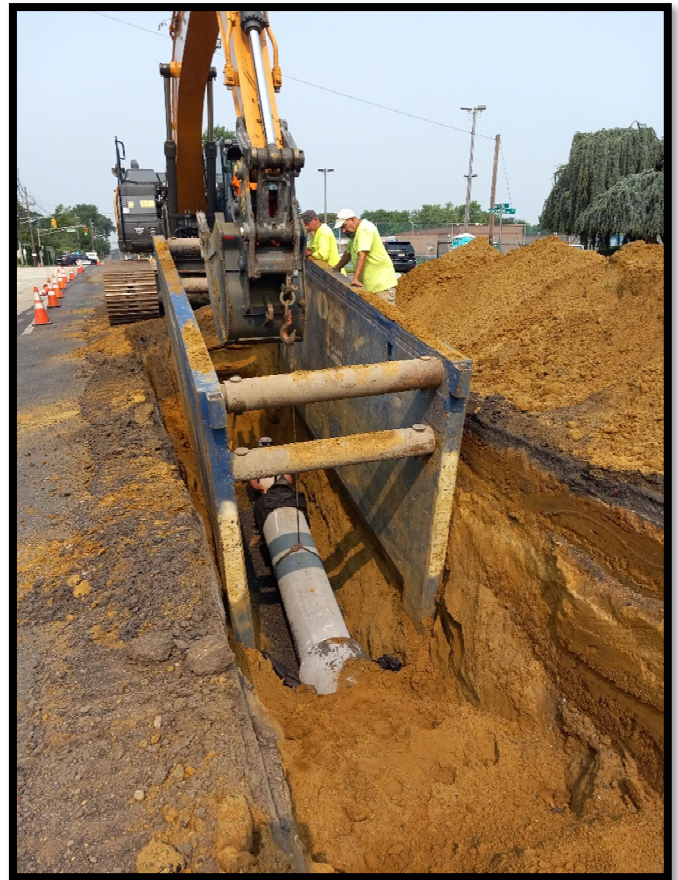
Photograph 2 – Pipe subcontractor installing 15" RCP storm pipe.
