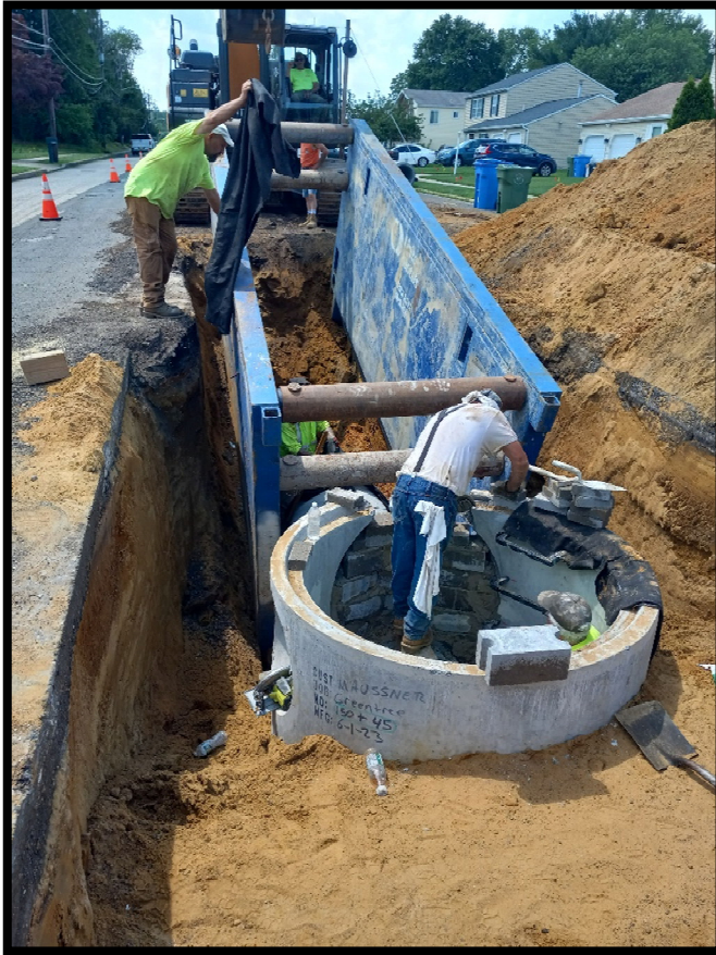
Photograph 7 –Manhole at Station 150+45 being installed.
