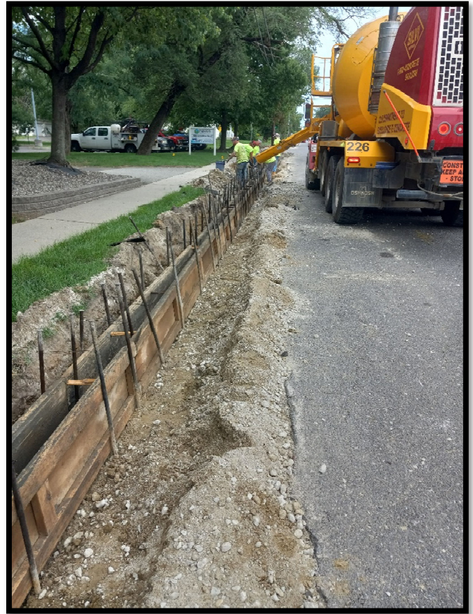
Photograph 2 – Concrete being place in forms for installation of concrete vertical curb.
