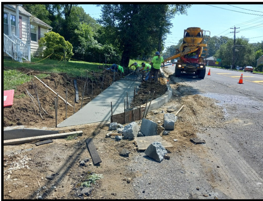
Photograph 4 – Concrete sidewalk being installed.
