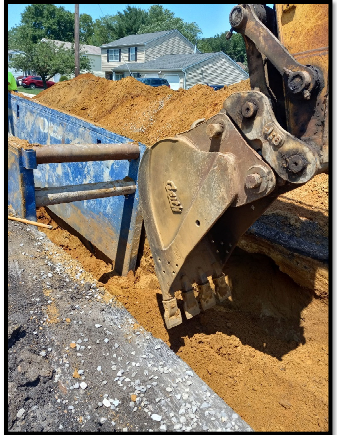
Photograph 8 – Excavating for installation of 30" RCP storm pipe.
