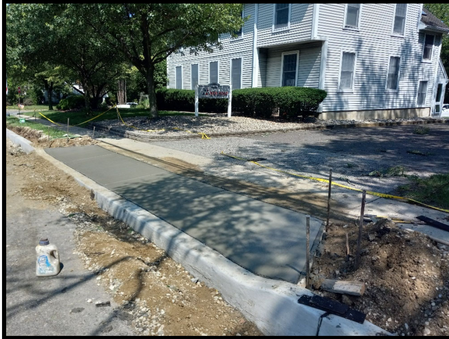
Photograph 5 – Concrete Driveway Apron after concrete pour.
