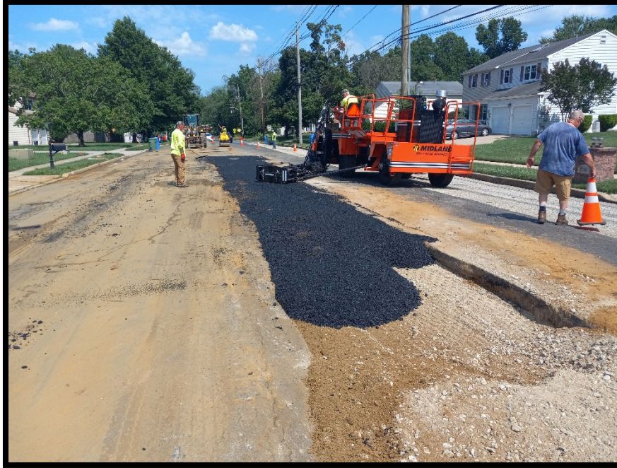
Photograph 9 – Asphalt trench restoration being completed after installation of 30" RCP storm pipe.
