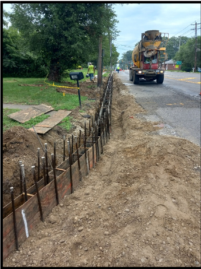
Photograph 1 – Curb forms set for installation of concrete vertical curb.
