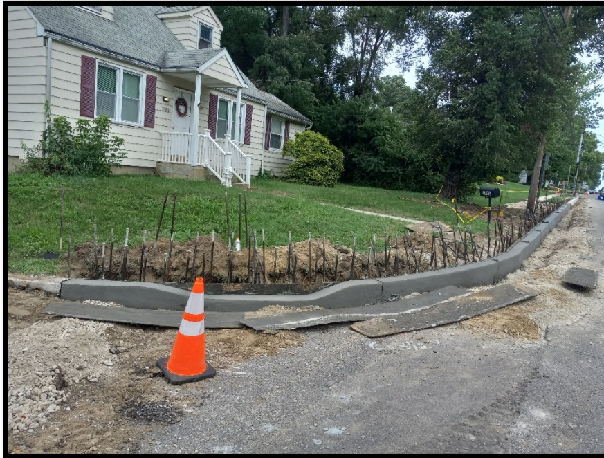
Photograph 3 – Concrete vertical curb after removal of forms.
