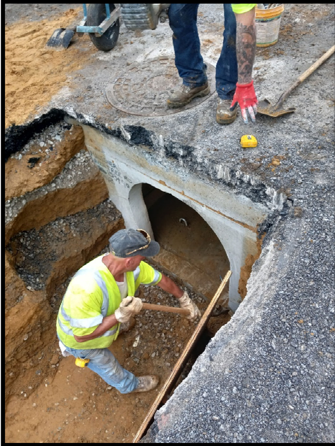
Photograph 5 –Preparing the trench for the 30” RCP at the diverter manhole.
