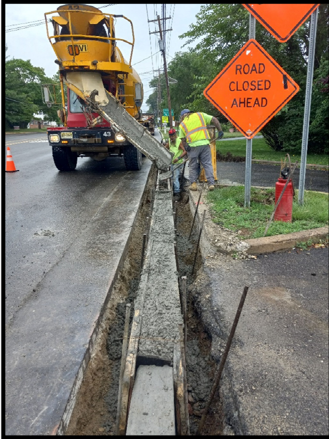
Photograph 7 – Concrete crew continued installing concrete curb between Route 70 and Springdale Road.
