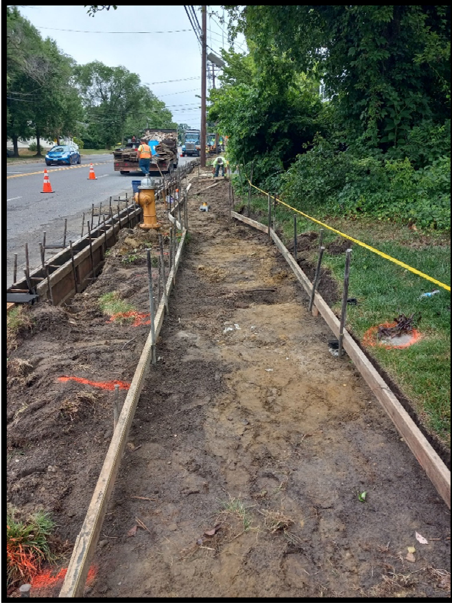
Photograph 5 – Curb and sidewalk forms installed in preparation of a concrete pour.
