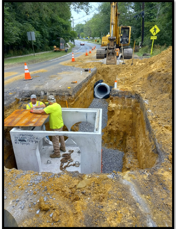
Photograph 4 – The pipe subcontractor installing the Diverter Manhole at Station 154+00.
