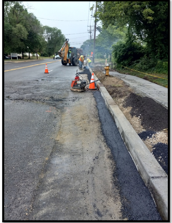
Photograph 6 – Asphalt restorations being completed after concrete curb is installed.
