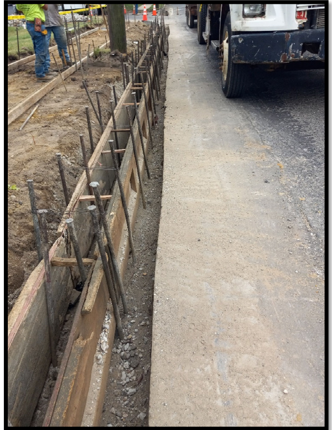
Photograph 4 – Curb forms installed in preparation of a concrete pour.
