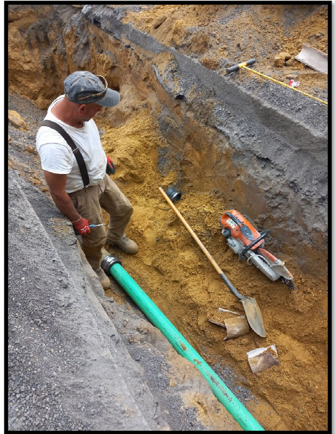
Photograph 2 – Permanent sewer lateral replacements completed at 1883 and 1887 Greentree Road.
