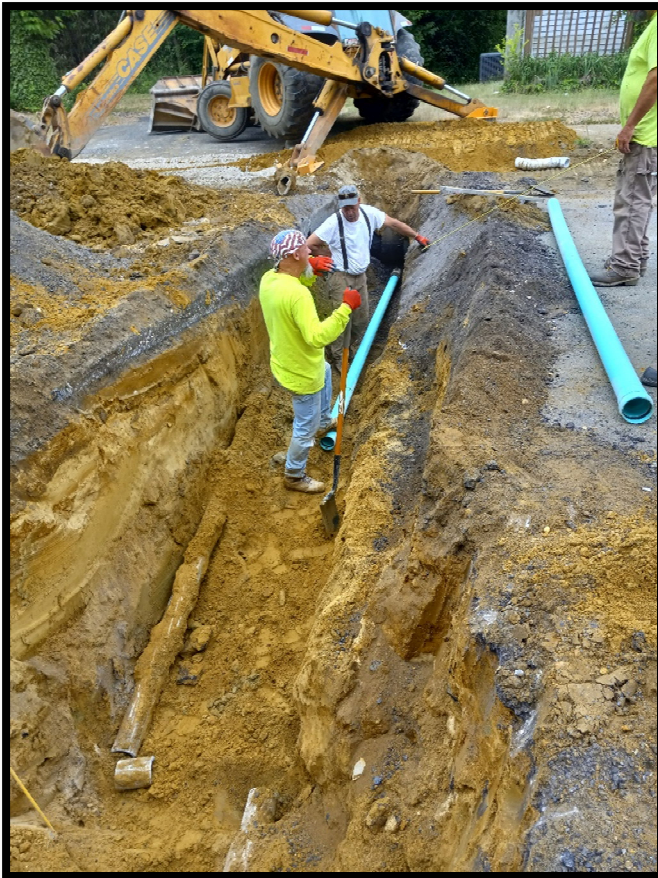
Photograph 1 – Permanent sewer lateral replacements completed at 1883 and 1887 Greentree Road.
