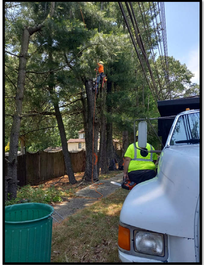
Photograph 4 – Tree removal subcontractor began removing trees per contract documents.
