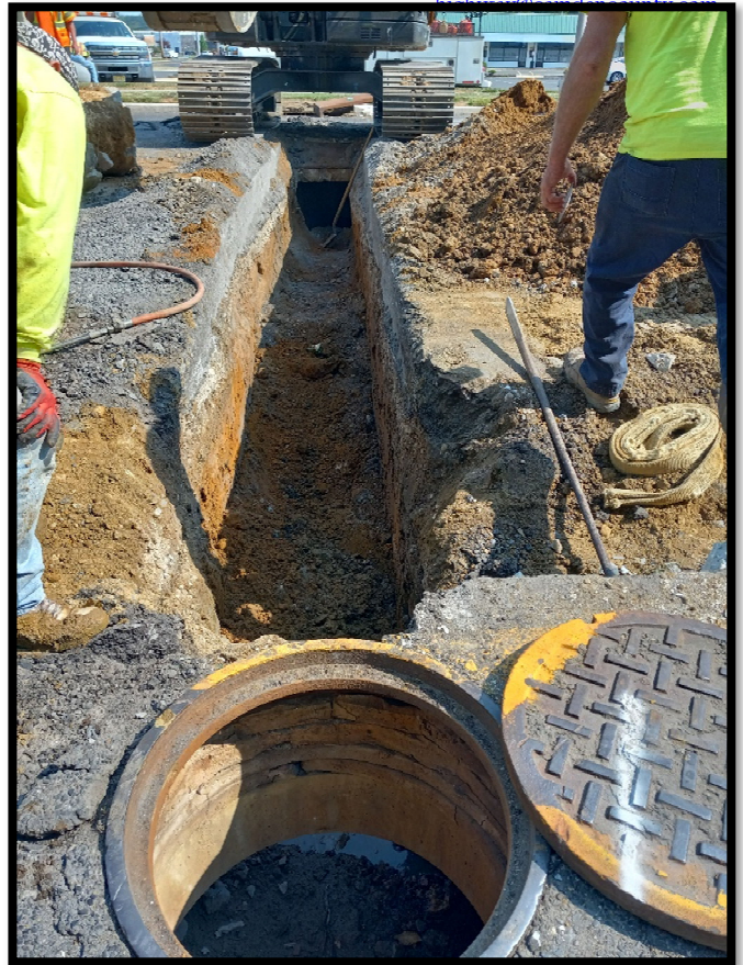
Photograph 8 – Trenching for 18" RCP cross drain at Station 118+00.
