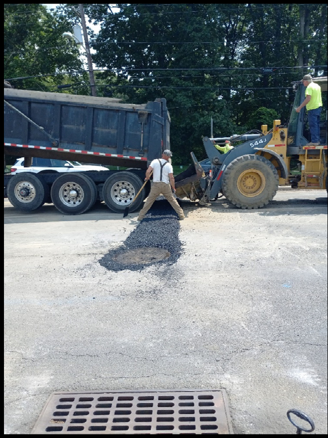
Photograph 9 – Temporary Asphalt Trench Restoration in progress for 18" RCP cross-drain at Station 118+00.
