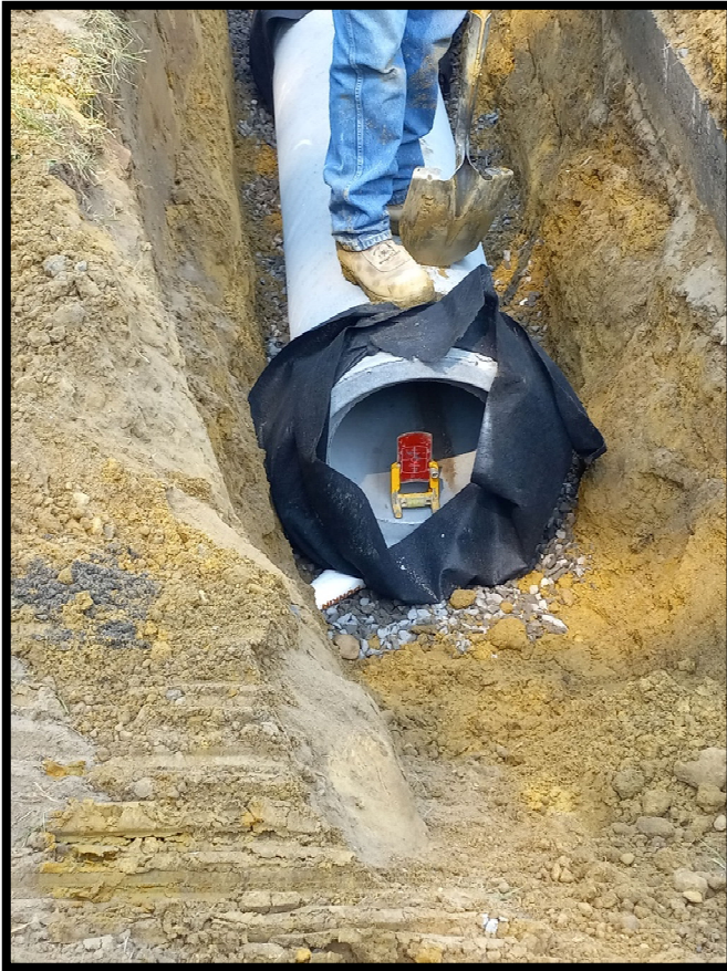
Photograph 3 – Laser level being utilized to ensure proper pitch of 15" Class 3 RCP.
