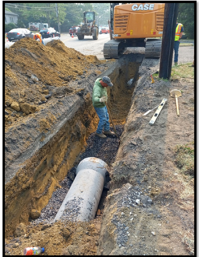
Photograph 2 – 15" Class 3 RCP being installed along the right side of Greentree Road.
