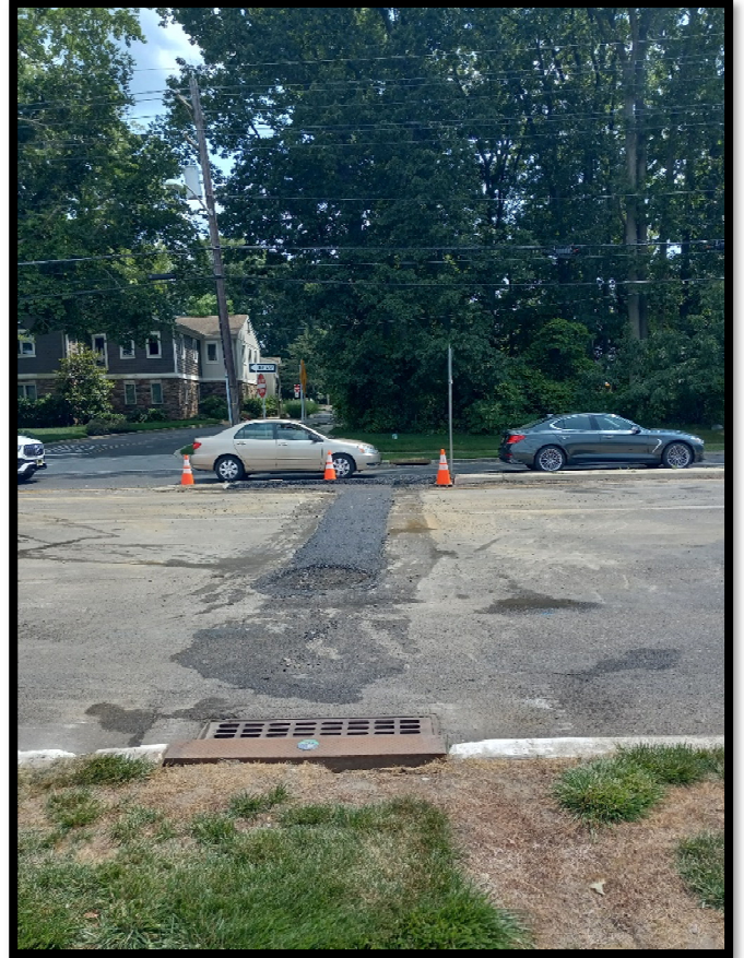
Photograph 10 – Temporary Asphalt Trench Restoration completed for 18" RCP cross-drain at Station 118+00.
