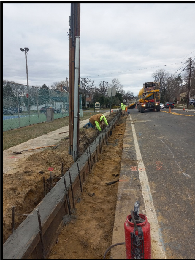
Photograph 1 – Curb being installed in front of Cooper Elementary School tennis courts.
