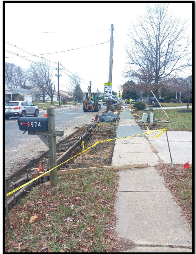
Photograph 2 – Preparing for Concrete Apron pour at 1974 Greentree Road.
