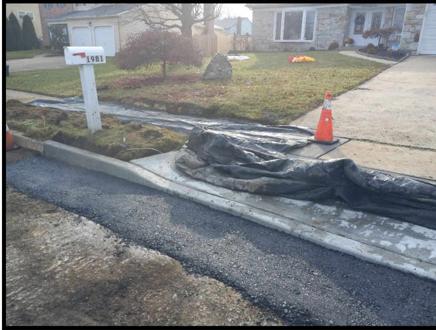
Photograph 7 – Asphalt restorations complete at curb installation for driveway at 1981 Greentree Road.
