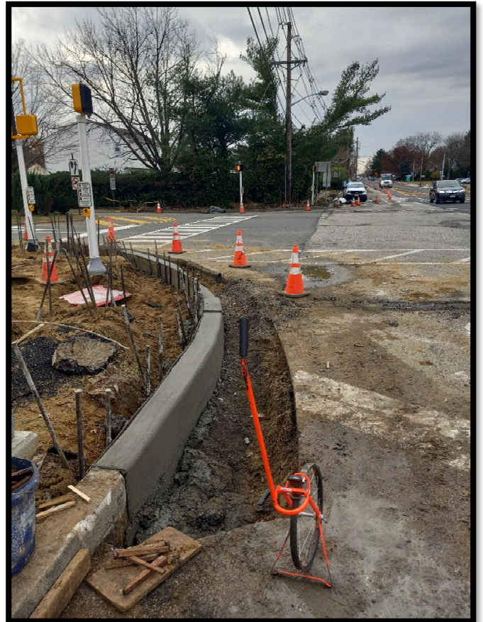
Photograph 2 – New concrete curb installed at the S. Birchwood Park Drive intersection.
