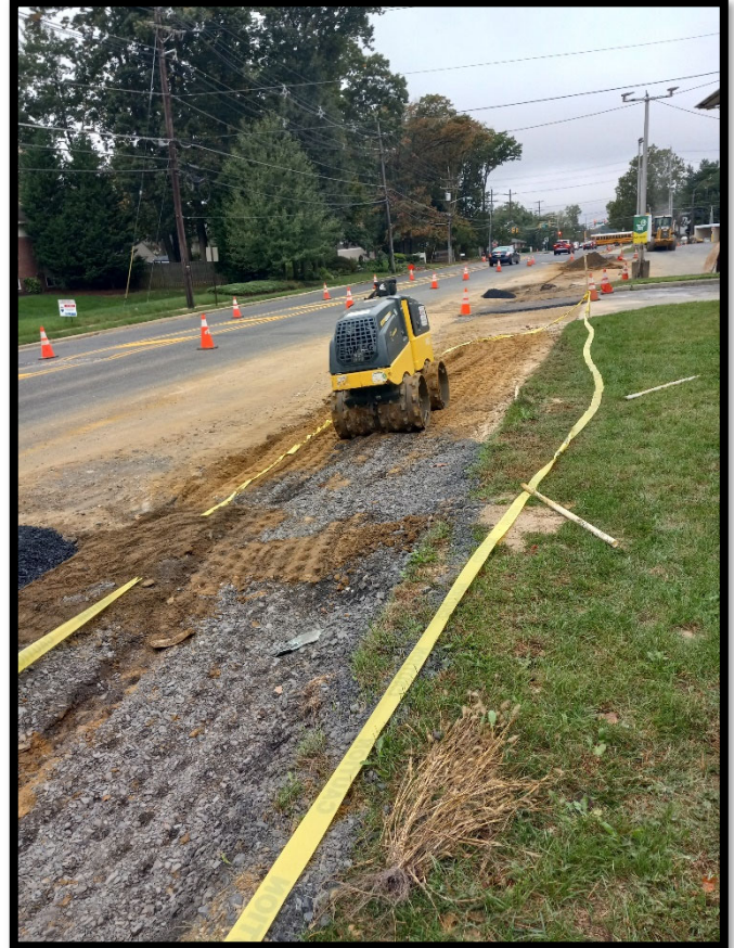
Photograph 4 – Pipe subcontractor preparing subbase for temporary sidewalk.
