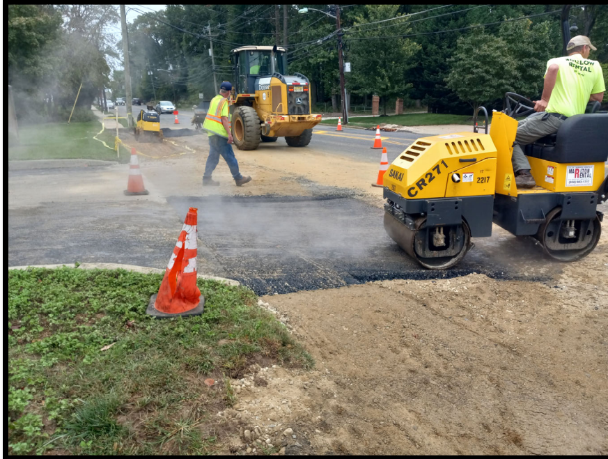
Photograph 7 – Temporary asphalt driveway apron being installed at 1926 Greentree Road.
