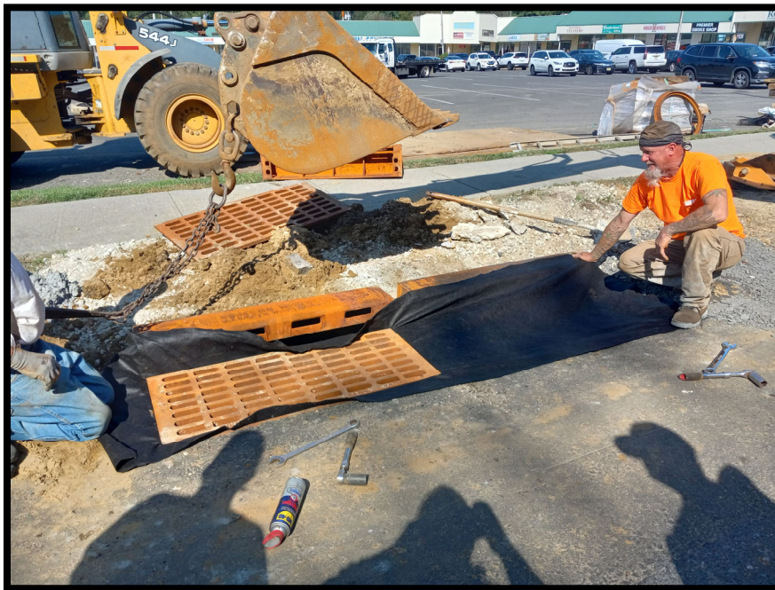
Photograph 6 – Inlet filters being installed to collect silt from roadway runoff.
