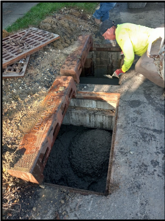
Photograph 1 – Pipe subcontractor installing concrete flow channels in the new 'B' inlets.
