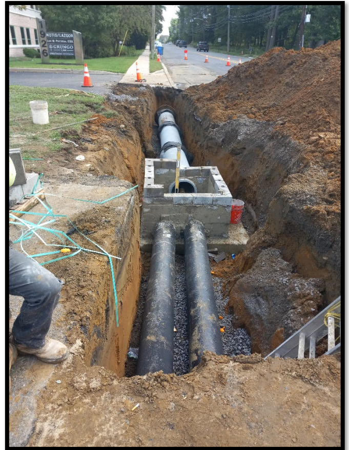
Photograph 2 – block work for 'B' inlet at Station 121+80L being installed.
