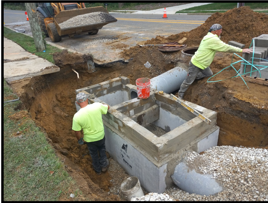
Photograph 5 – Inlet block being installed at Double 'B' inlet at Station 122+75L.
