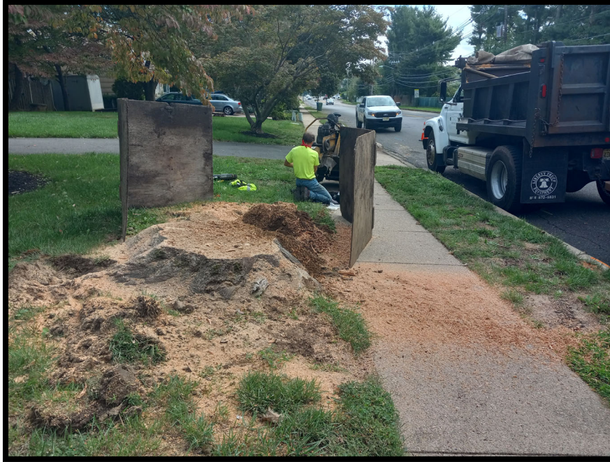
Photograph 7 – Tree subcontractor preparing to grind stump at Station 131+00L.
