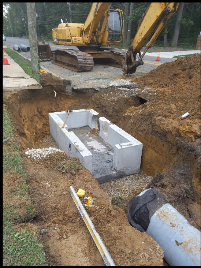
Photograph 3 – Double 'B' inlet being installed at Station 122+75L.
