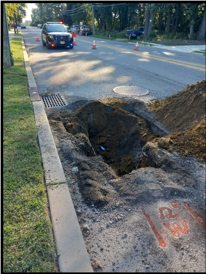
Photograph 1 – Pipe subcontractor digging test pits near Station 122+75 to locate existing 12” watermain.
