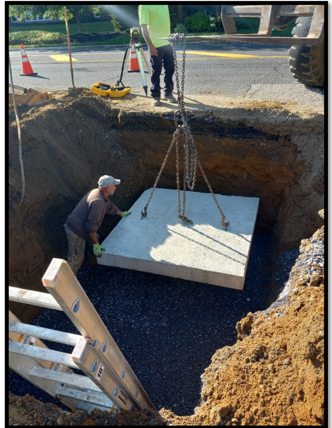
Photograph 2 – Precast slab being installed for “B” Inlet at Station 120+75L.
