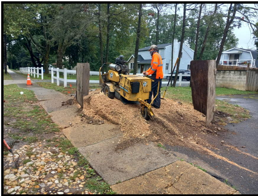
Photograph 6 – Tree subcontractor grinding stump at Station 127+75L.
