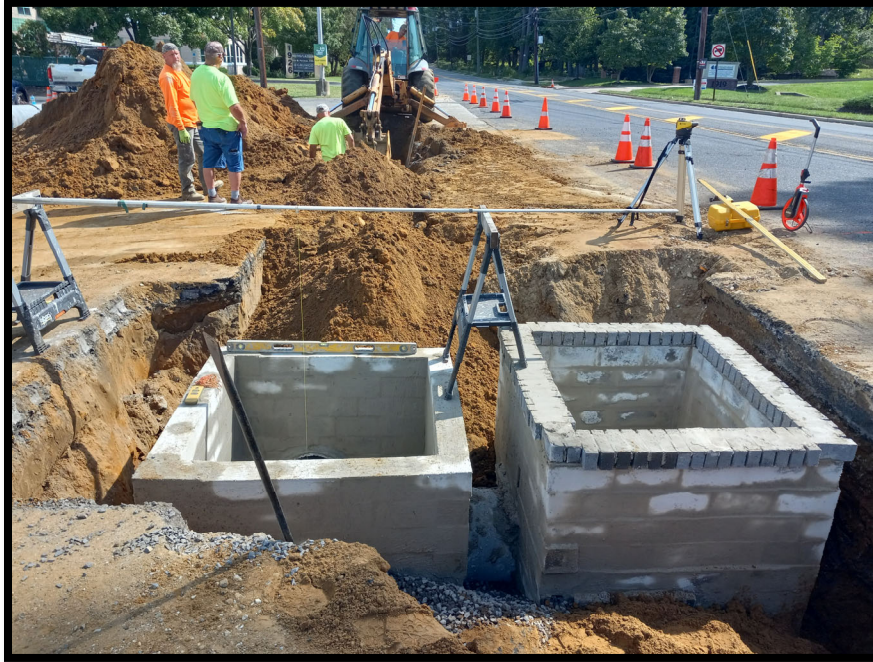
Photograph 5 – “B” inlet on right and manhole on left at Station 120+75L.
