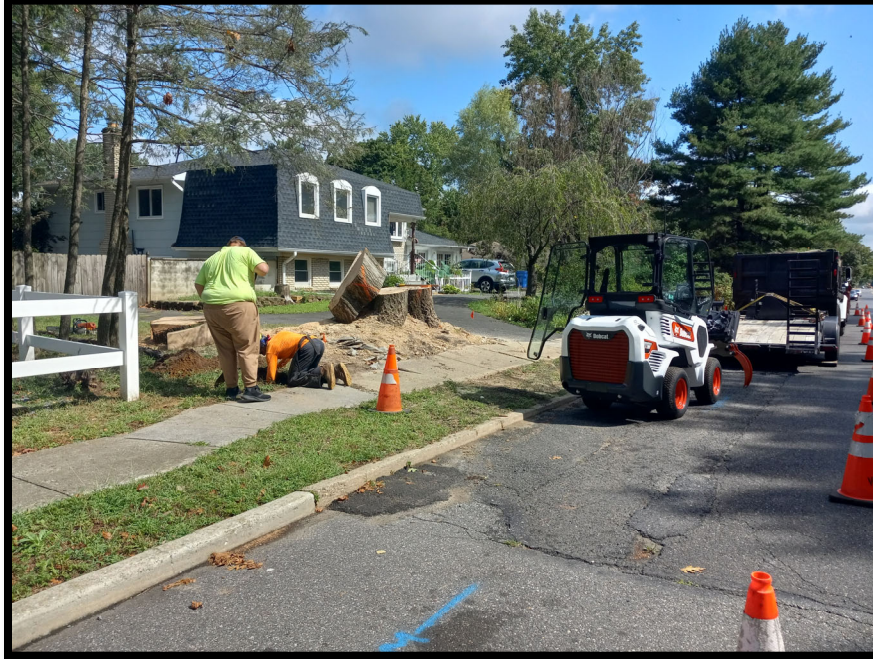
Photograph 5 – Tree subcontractor preparing to grind stumps at Station 127+75L and 128+75L.
