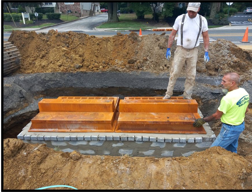
Photograph 5 – Pipe subcontractor installing new Double “B” Inlet Castings at Station 118+90L.
