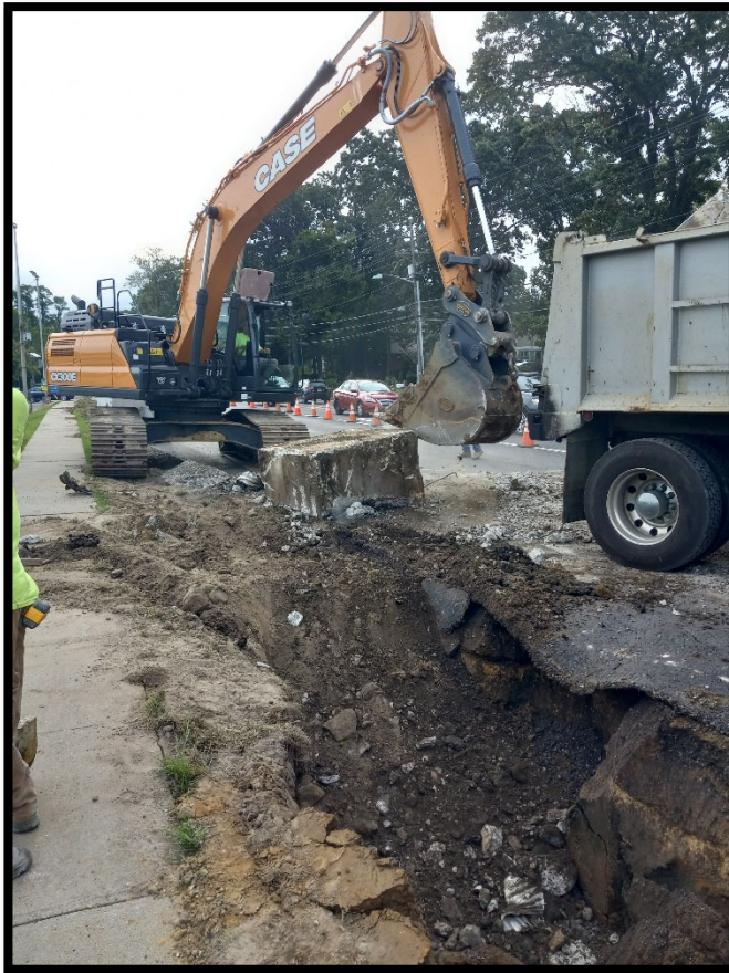
Photograph 1 – Pipe subcontractor demolishing existing inlet at Station 118+00L.
