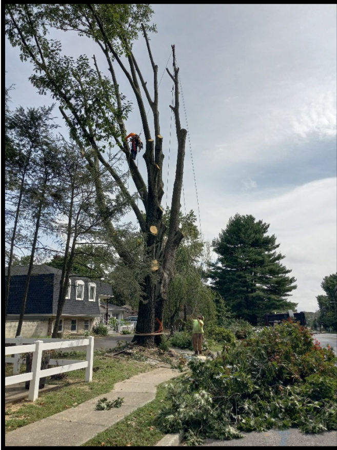
Photograph 3 – Tree subcontractor removing tree at Station 127+75L.
