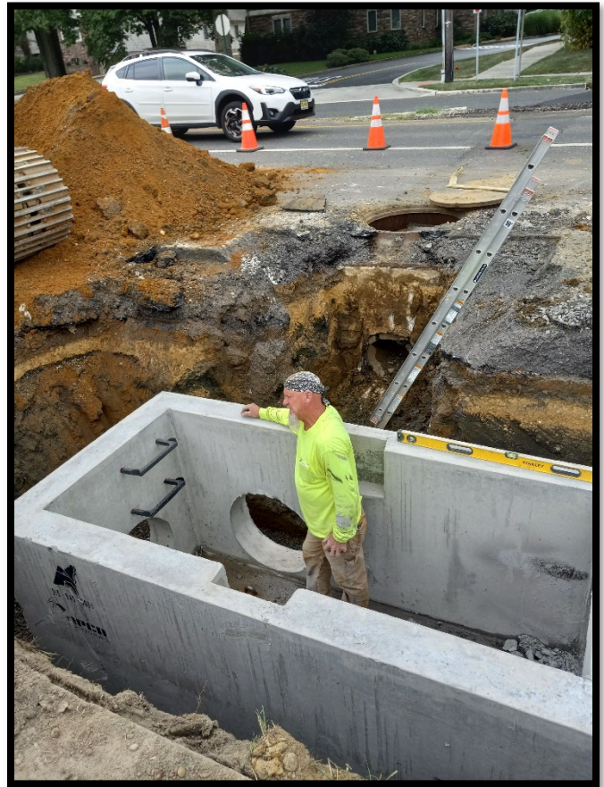
Photograph 2 – Pipe subcontractor installing new Double "B" inlet at Station 118+00L.
