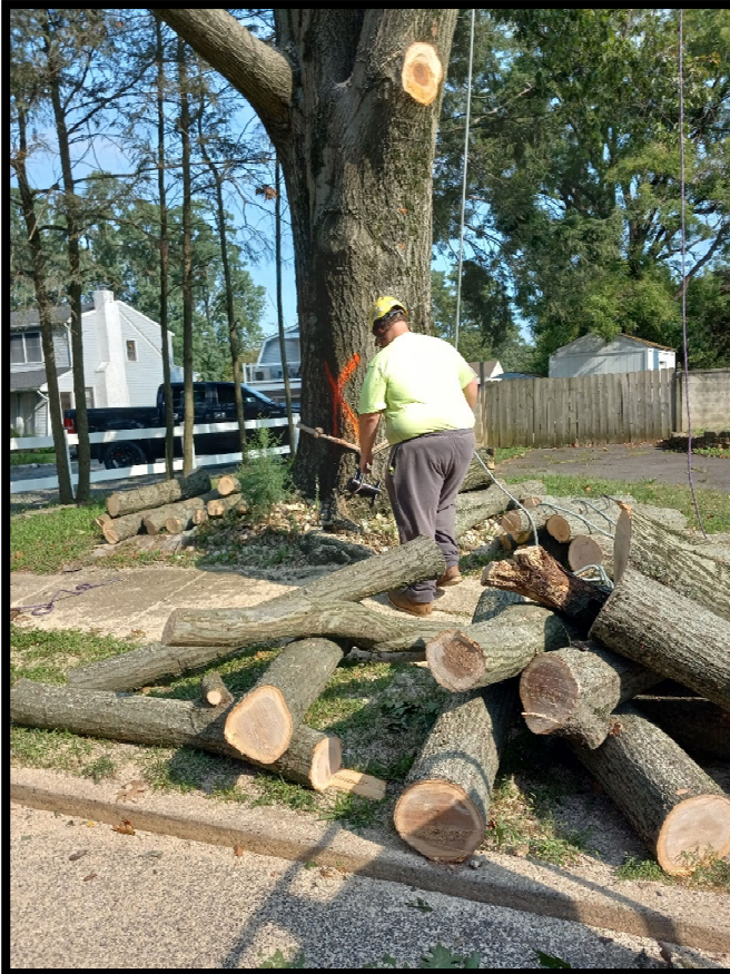
Photograph 2 – Tree subcontractor removing the tree at Station 127+75L.
