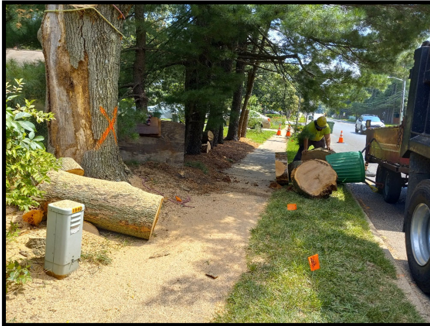
Photograph 6– Tree subcontractor removing tree at Station 128+75L.
