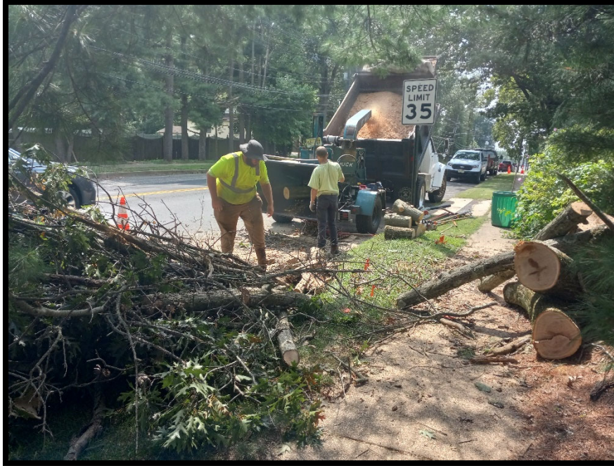
Photograph 3– Tree subcontractor removing trees at Stations 131+00L and 128+75L.
