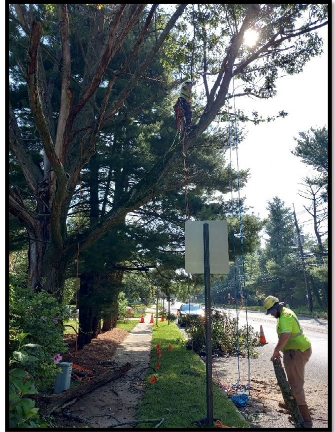
Photograph 2 – Tree subcontractor removing trees at Stations 131+00L and 128+75L.
