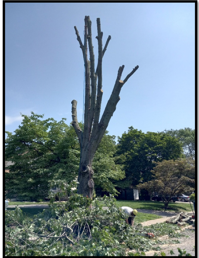
Photograph 5 – Branches removed in preparation of tree removal at Station 131+00L.
