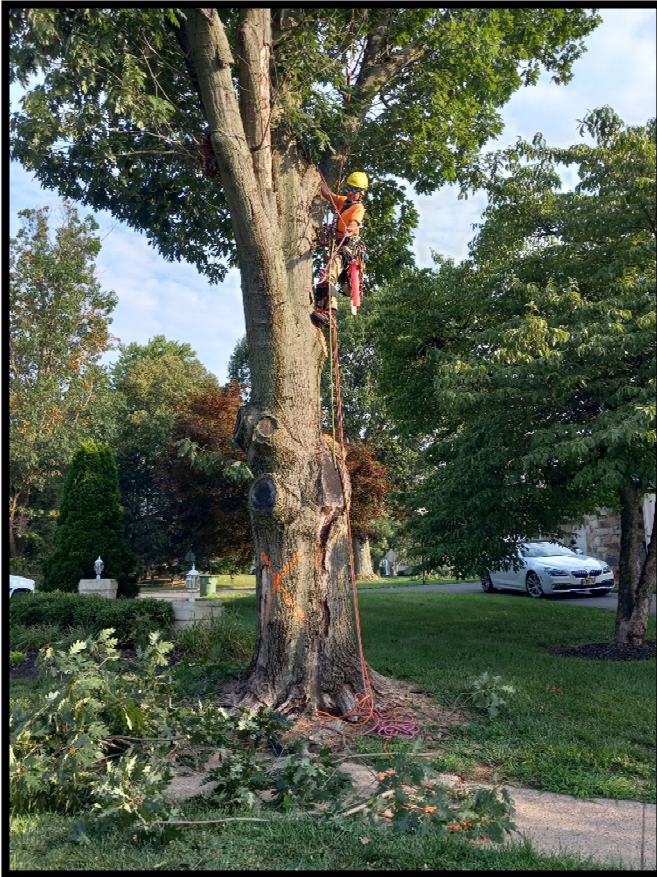
Photograph 4 – Tree subcontractor removing branches for tree removal at Station 131+00L.
