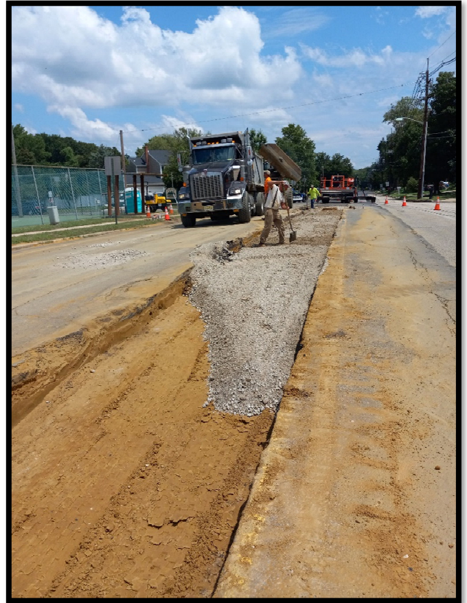
Photograph 3 – Trench restoration after installation of 15” RCP storm pipe.
