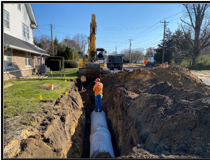
Figure 3: P&A Construction installing reinforced concrete pipe.
