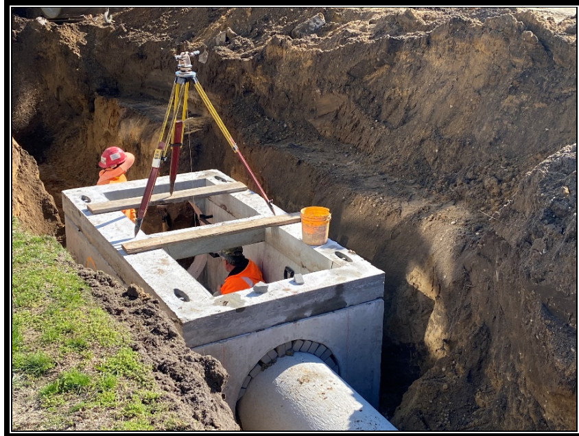
Figure 2: P&A Construction installing precast concrete structures.
