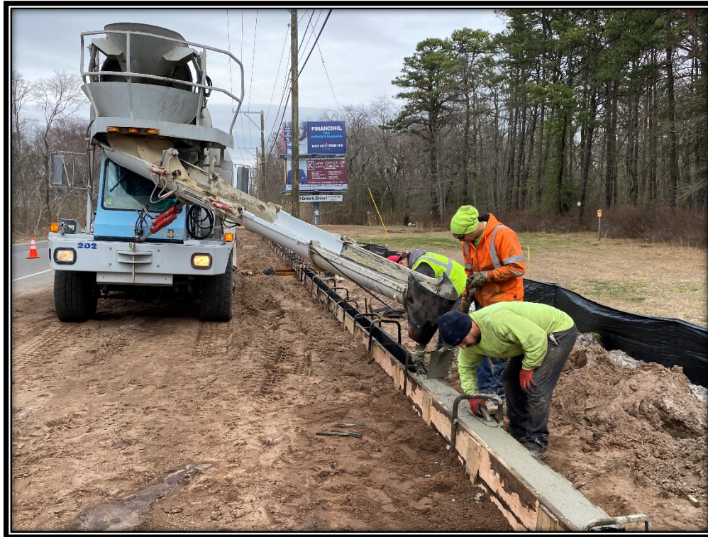
Figure: P&A Construction started the 9"x18" concrete vertical curb.
