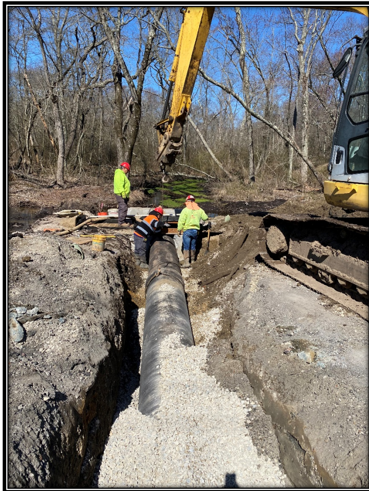
Figure: P&A Construction installing ductile iron pipe crossing.
