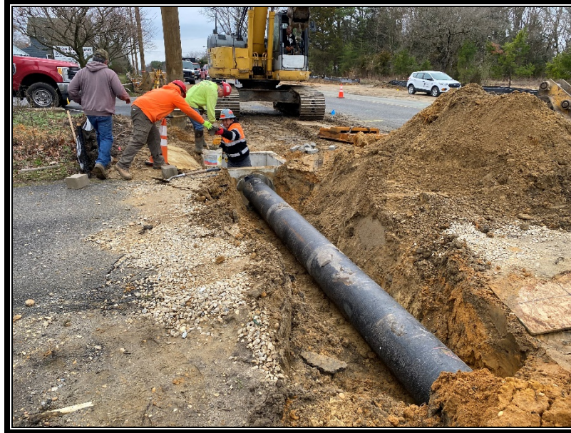
Figure 2: P&A Construction installing ductile iron storm pipe.
