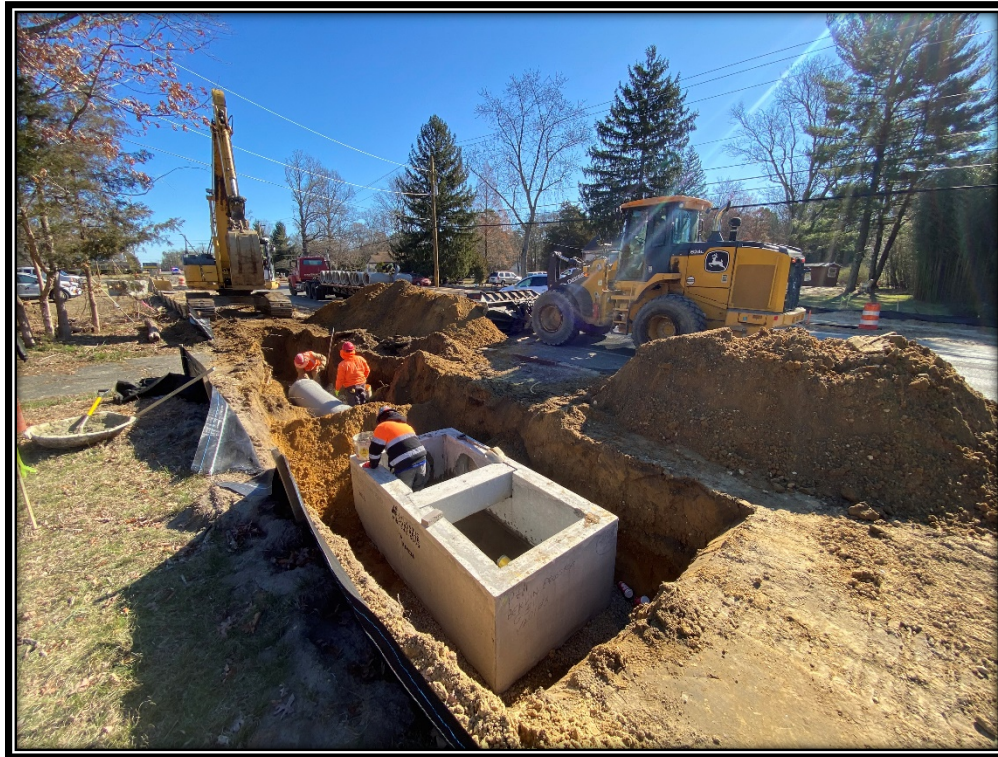
Figure: P&A Construction installing reinforced concrete structures.
