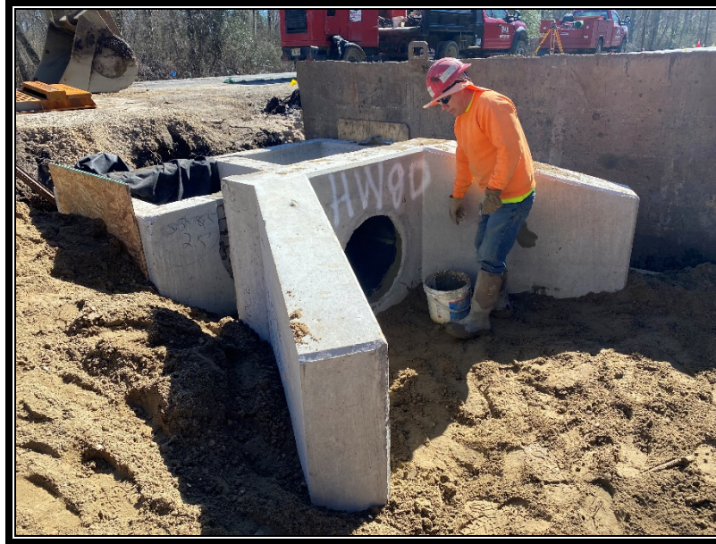
Figure 2: P&A Construction installing precast concrete headwalls.
