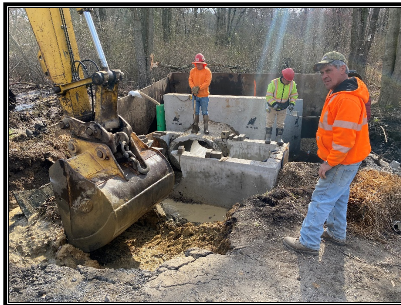
Figure 3: P&A Construction installing precast concrete structures.
