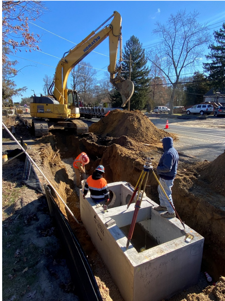
Figure: P&A Construction installing reinforced concrete structures.
