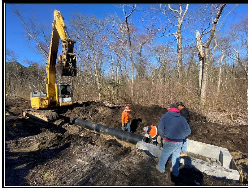
Figure 2: P&A Construction installing ductile iron pipe.
