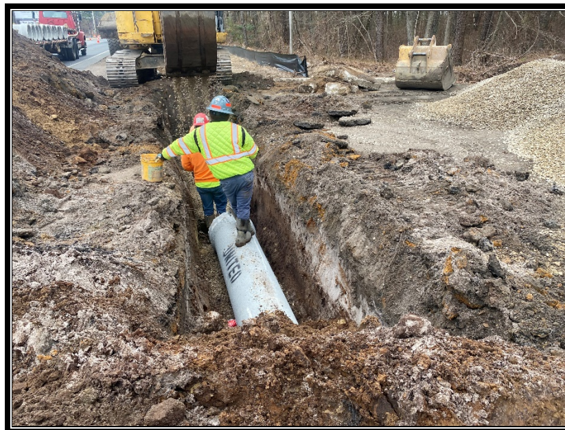
Figure 3: P&A Construction installing reinforced concrete pipe.
