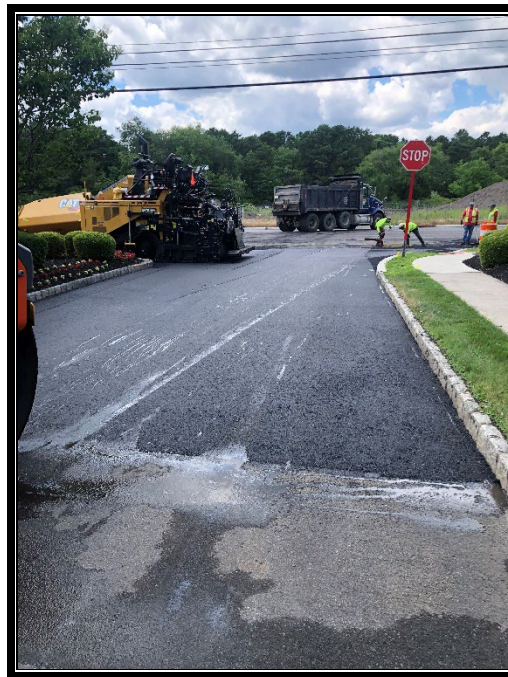
Figure 3: P&A Construction paves HMA surface course.
