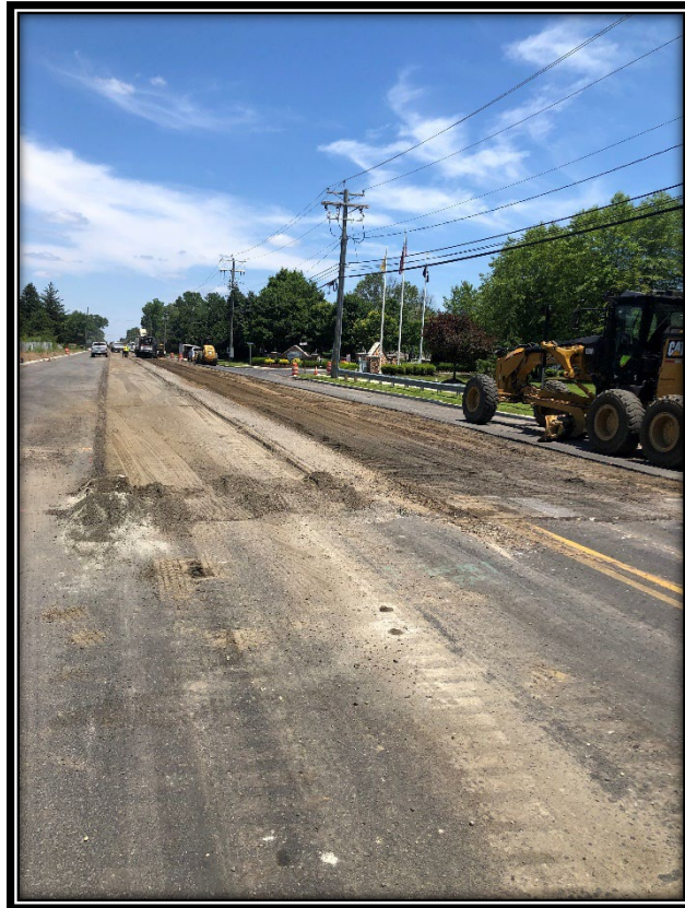
Figure:1 Full depth pavement reclamation from Madison to Franklin.
