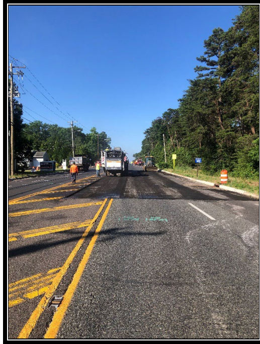
Figure 2: Milling for final surface course.
