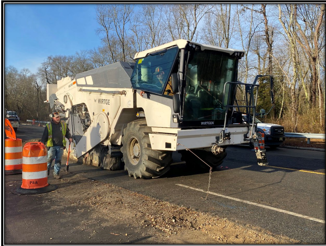
Figure:1 Asphalt Paving Systems, mobilizing Full Depth Pavement Reclamation equipment.
