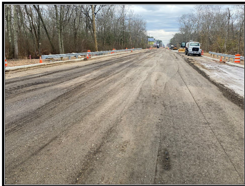
Figure 3: Asphalt Paving Systems pulverizing the existing pavement.
