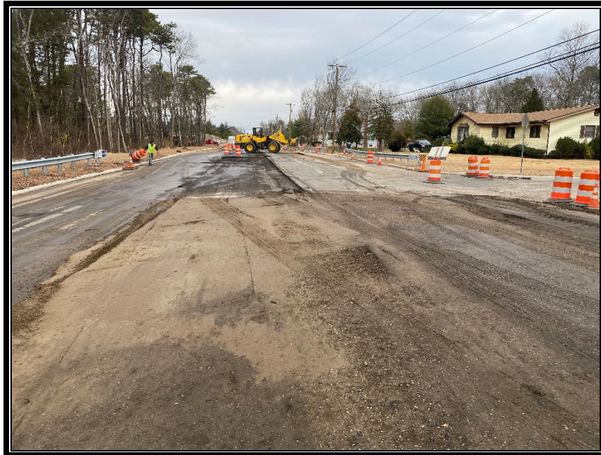
Figure 2: P&A Construction starting to mill existing roadway surface
