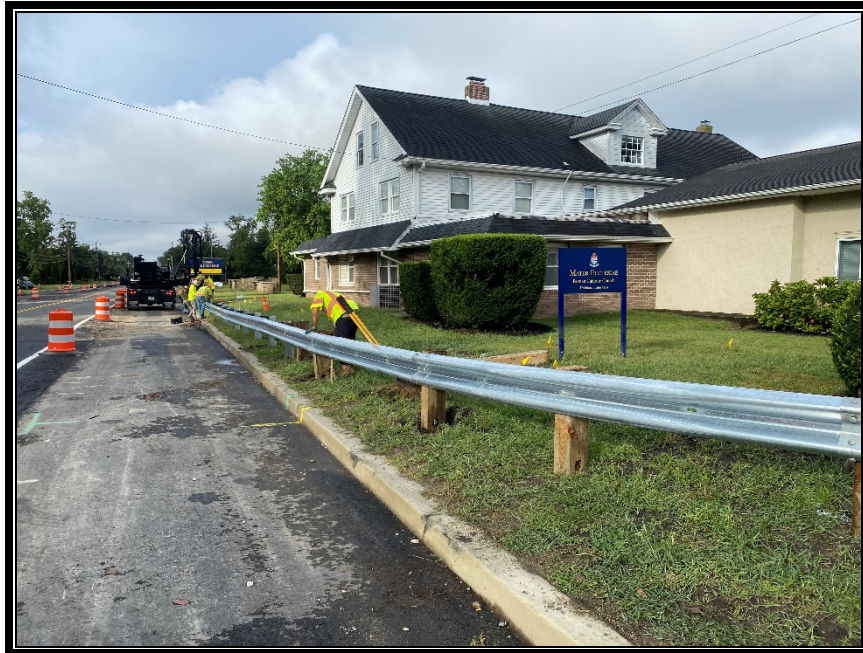
Figure 2: RSS Roadway Safety Systems, LLC installing guide rail and end treatments.
