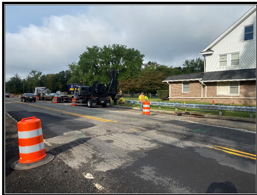
Figure 3: RSS Roadway Safety Systems, LLC installing guide rail and end treatments.
