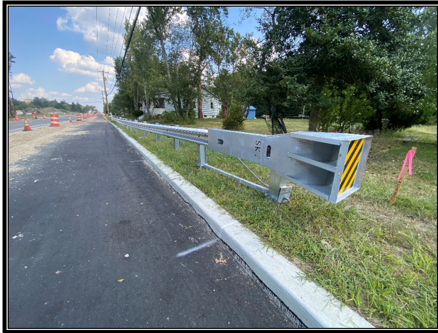
Figure 2: RSS Roadway Safety Systems, LLC installing guide rail and end treatments.
