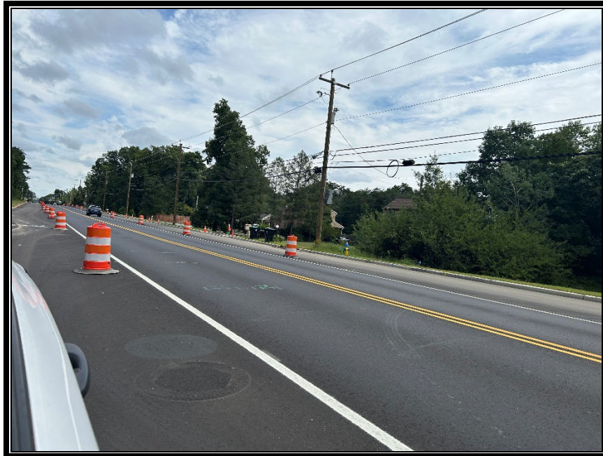
Figure 2: P&A Construction maintains traffic control during project shutdown.
