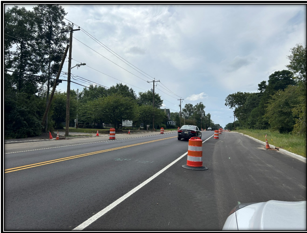
Figure: P&A Construction maintains traffic control during project shutdown.
