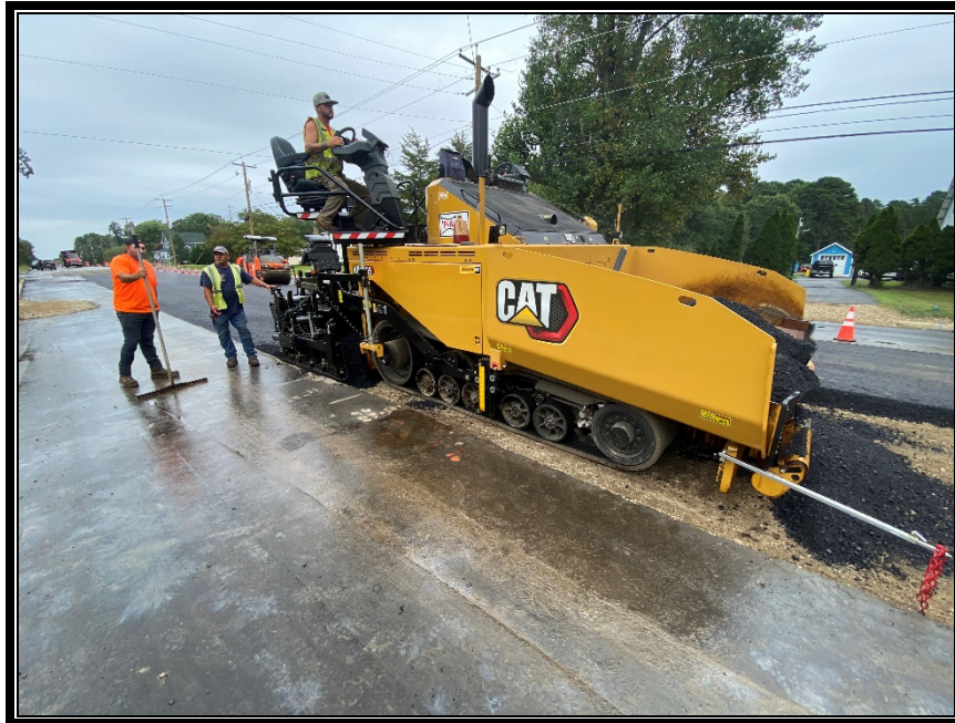
Figure 2: P&A Construction continues to pave the base course asphalt.
