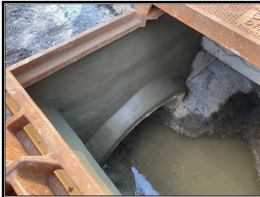
Figure 3: P&A Construction continues to parge inlets and manholes.
