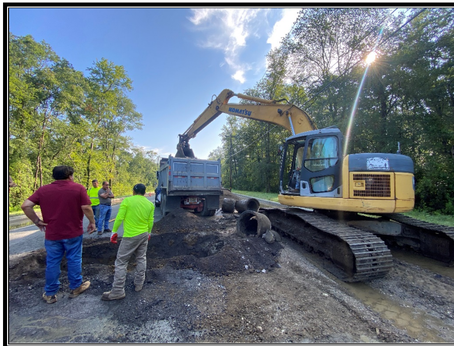
Figure 3: P&A Construction removing an existing 24" R.C.P.
