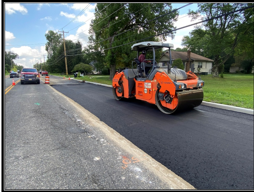
Figure 2: P&A Construction using a roller to ensure proper compaction.
