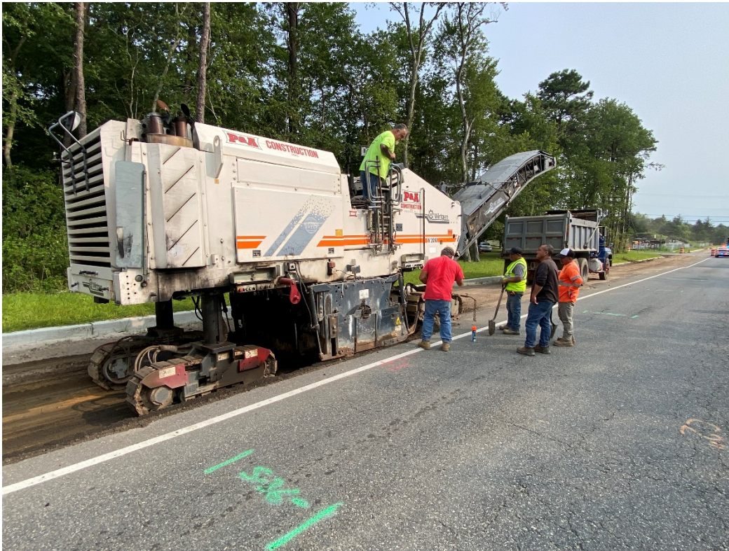
Figure: P&A Construction continues to excavate using the milling machine.
