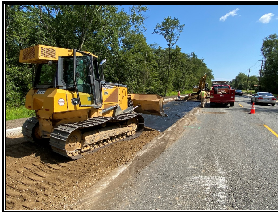
Figure 3: P&A Construction continues to construct the widening.
