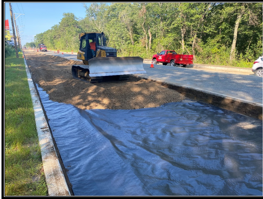
Figure 2: P&A Construction continues to install the roadway stabilization fabric and D.G.A.
