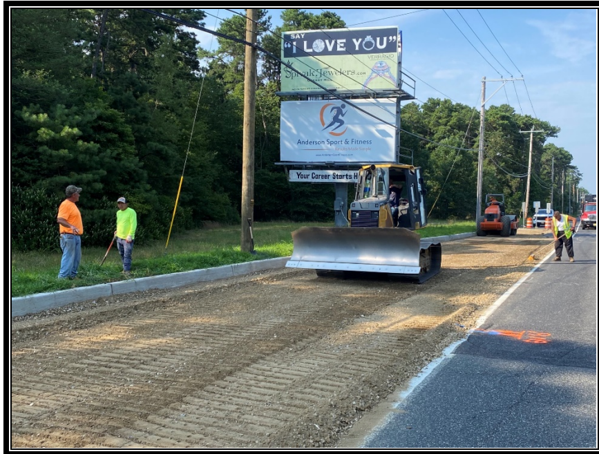
Figure 2: P&A Construction continues to excavate and install dense graded aggregate.
