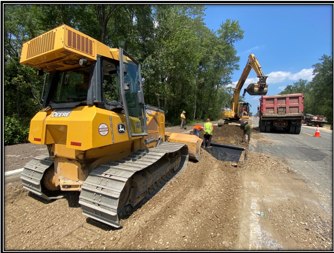
Figure: P&A Construction continues to excavate and install dense graded aggregate.
