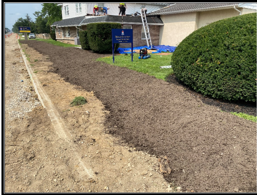
Figure 2: P&A Construction continues to install topsoil, seed and fertilizer.
