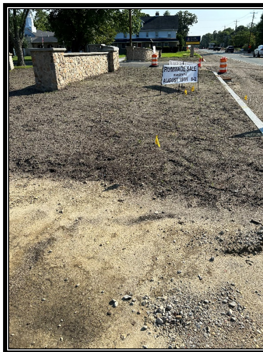
Figure 3: P&A Construction continues to install topsoil, seed and fertilizer.
