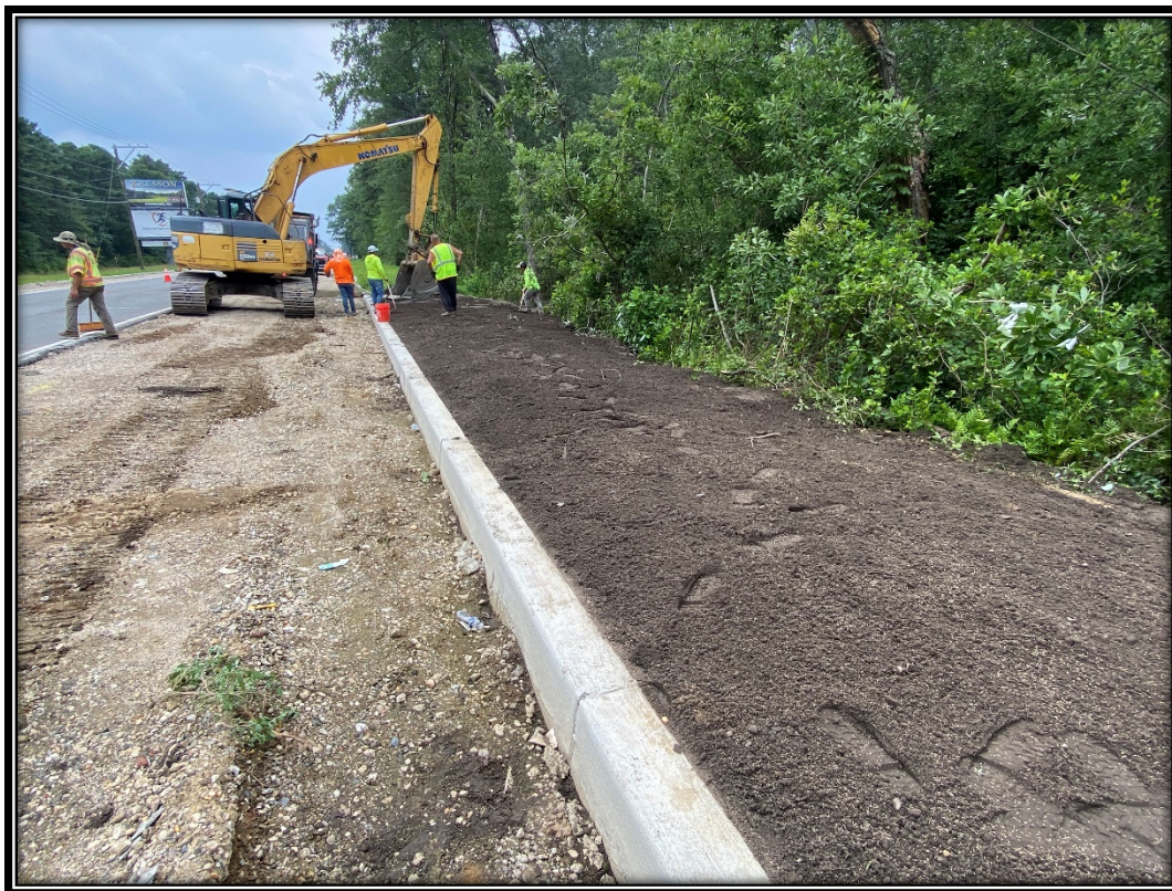
Figure: P&A Construction continues to install topsoil, seed and fertilizer.
