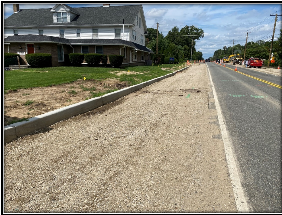
Figure: P&A Construction continues to install Dense Graded Aggregate.
