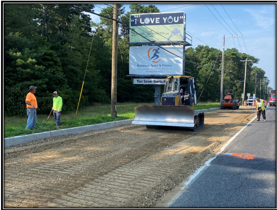
Figure: P&A Construction excavated roadway and installed DGA Base Course.
