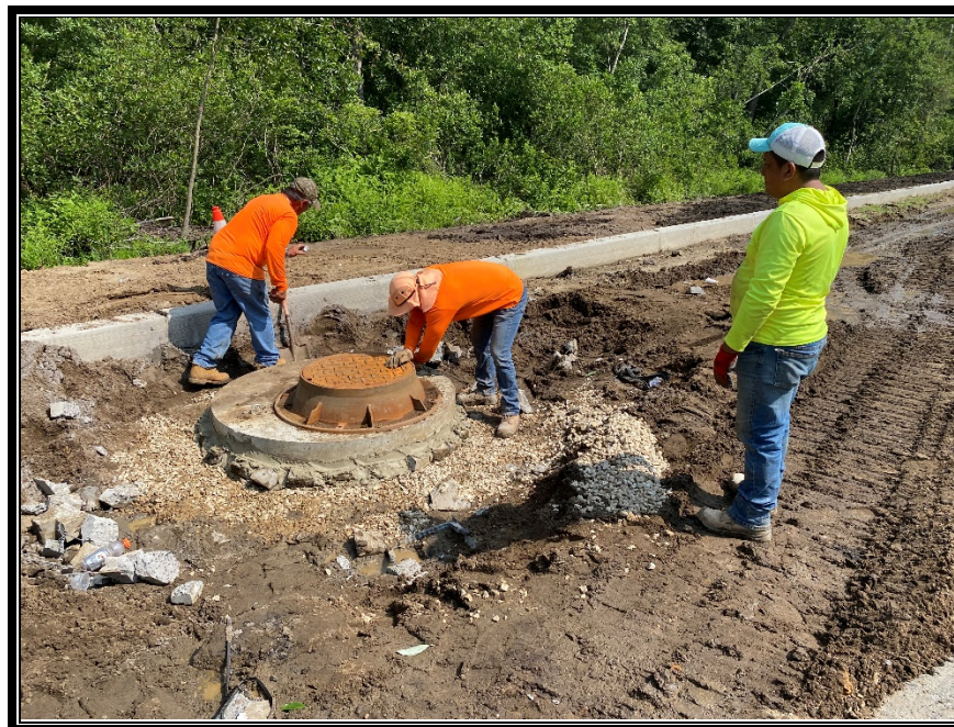
Figure 3: P&A Construction set drainage structures to finished grade.
