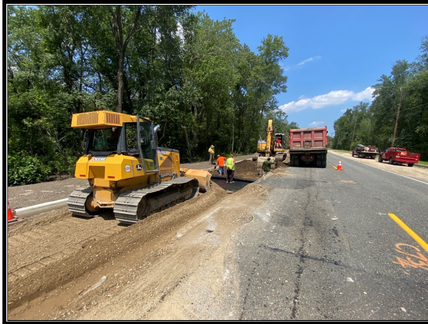
Figure 2: P&A Construction excavated roadway and installed DGA Base Course.
