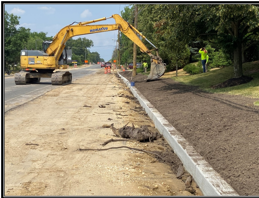
Figure 3: P&A Construction continues to install topsoil, grass seed and fertilizer.
