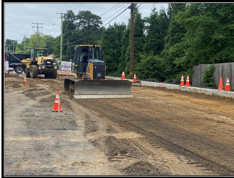
Figure 2: P&A Construction started grading the sub-grade for the roadway.
