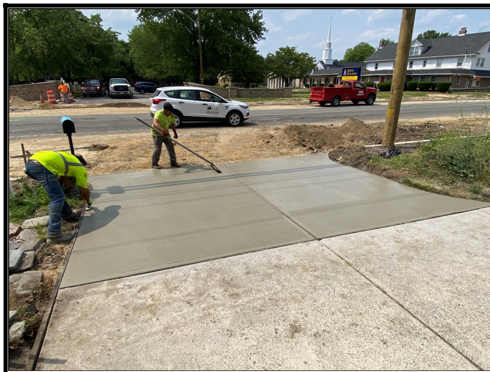
Figure 3: P&A Construction forming and pouring concrete aprons.
