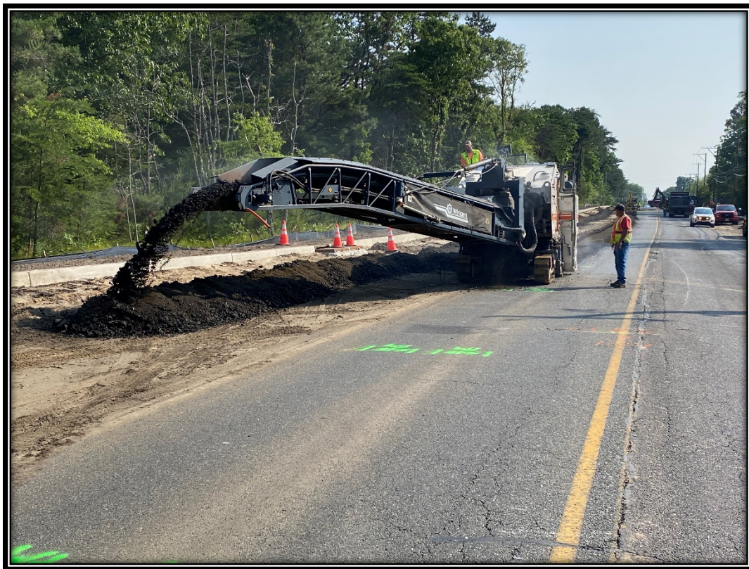
Figure: P&A Construction started to mill out the existing asphalt roadway.
