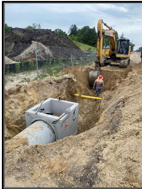
Figure 3: P&A Construction continues to install the new R.C.P. and inlets.
