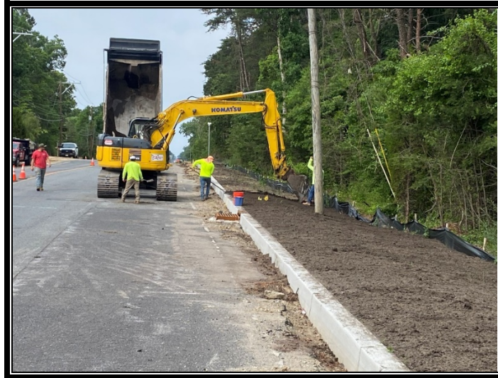
Figure 2: P&A Construction started to install the topsoil, fertilizer and grass seed.
