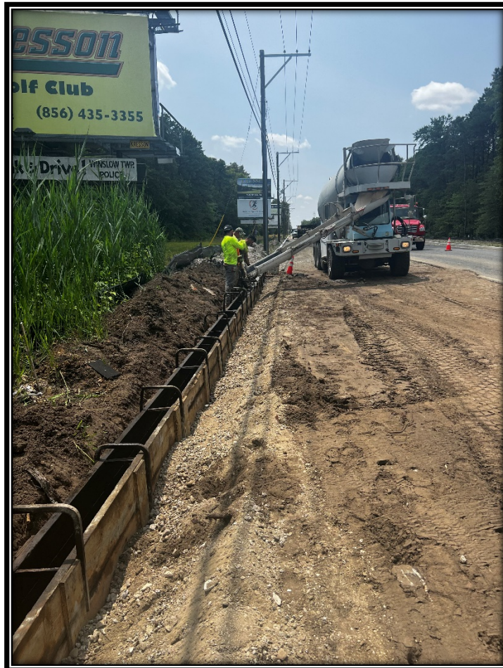
Figure: P&A Construction continues to install concrete vertical curb.
